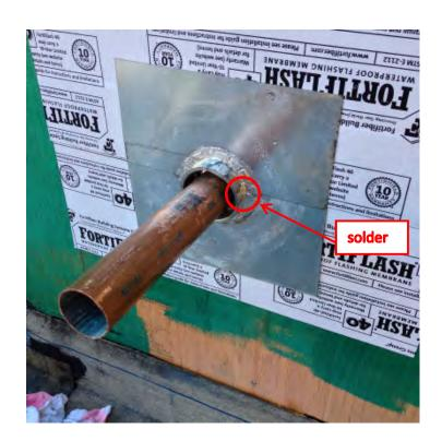
Install 2-piece pipe collar flashing, with 4" min. lap set in a full bed of sealant and secured to substrate with "S.S. Pan-Head screws" or "hot-dip galvanized nails" as required.
