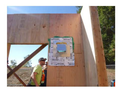
Install fully-soldered wall cap with insect screen into R.O. with "S.S. pan-head screws" or "hot-dip galvanized nails".
