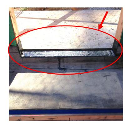
Confirm podium waterproofing installed onto door sill pan and up jambs **prior** to door frame installation.
