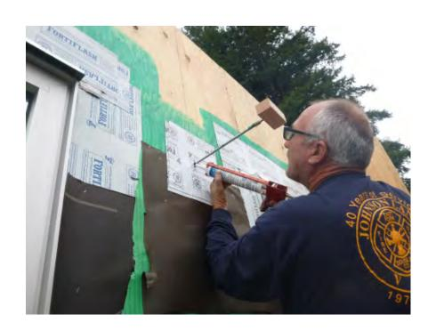
Apply sealant all around bolt (Step 4)
