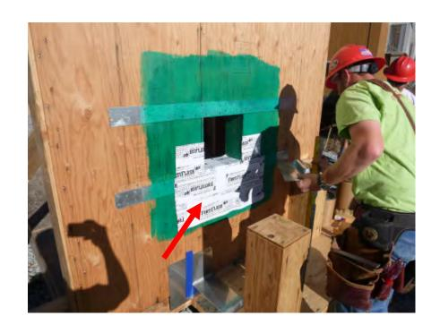
Install SAF along sill of wall cap opening with release paper remaining on bottom half of SAF or provide starter strip of WRB prior to SAF installation.
