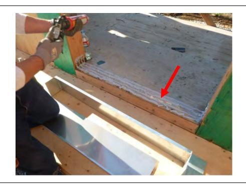
Sealant applied along door sill and wall flanges for sill pan installation.
