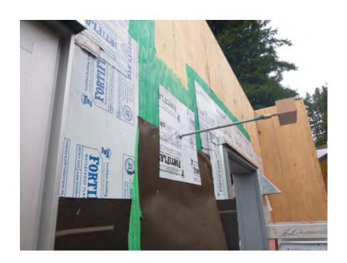
Apply SAF "sill" at bolt over WRB starter strip and sheathing. (Step 2)
