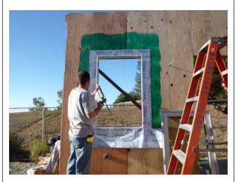
Apply continuous bead of Silicone or Moistop sealant at window head and jamb sides.
