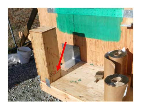
Column kerf cut location to be determined by topping slab height. Existing may be acceptable. Extend cut around entire perimeter of column.
