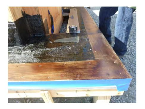
Set 22 GA S.S. edge metal into WP membrane, fastened @ 4" o.c., 2-rows staggered.
