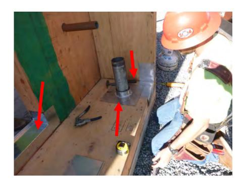
Prior to installation of podium WP confirm preceding installations complete (i.e. sheet metal saddles, door sill pans, continuous wall flashing, etc).
