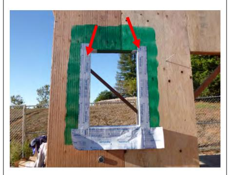
12" wide SAF installed along jamb over sheathing face 4" and extending 4" beyond rough opening @ top & bottom.
