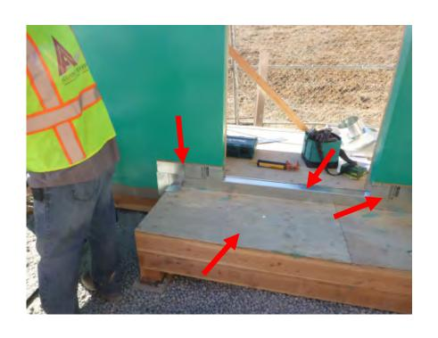
PRIMER is to be applied using a <u>hand</u> <u>held sprayer</u> onto **ALL** surfaces receiving the podium WP membrane.
