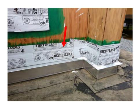
Install 9" wide SAF lapped over top leg of GSM weep screed.
