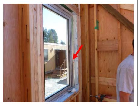
Install GSM angles along jambs, set in a full-bed of sealant.
