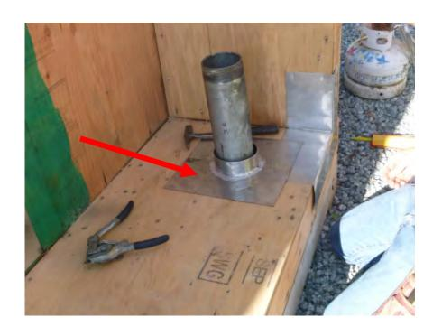
2-piece S.S. pipe collar, with hemmed top edge secured to deck w/ fasteners and sealant
