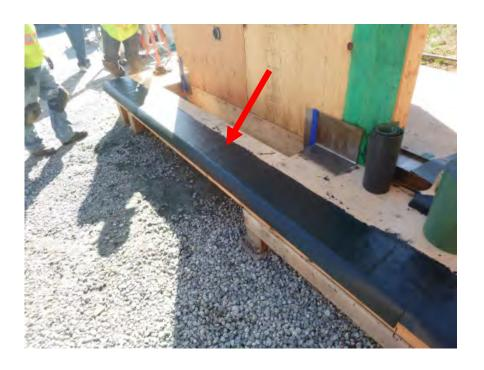
Set 9" wide uncured neoprene onto horizontal surface of edge allowing min 3" of neoprene onto vertical surface.
