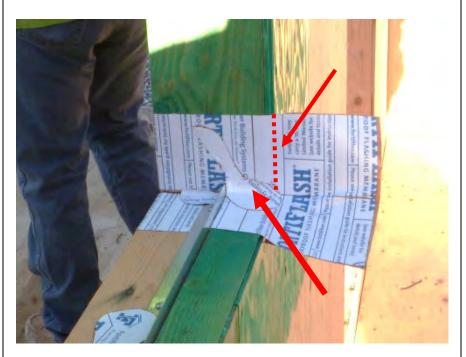
SAF butterfly patches installed at sill GSM angle to jamb intersections.
