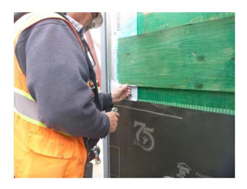
Primer applied onto stucco band surfaces to receive SAF.
