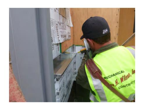
Set GSM flashing into full bed of sealant on top shelf of stucco band.
