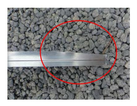
L-metal interlocking leg trimmed at base of door jambs to accommodate base flashing waterproofing build-up.
