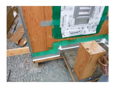
Install GSM weep screed at base of wall onto substrate with "S. S. Pan-Head screws" or "hot-dip galvanized nails".
