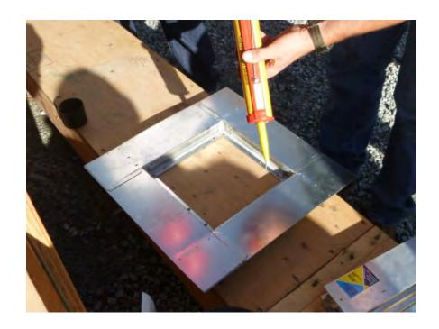
Apply sealant between nailing flange and louver
