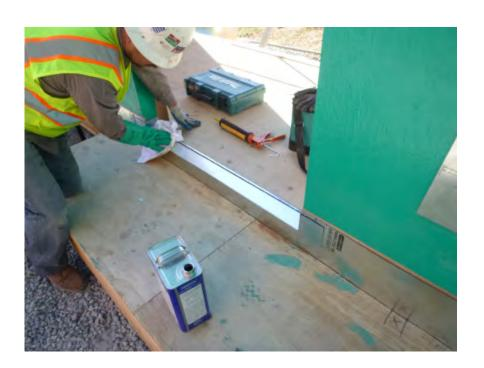
Clean the substrate(s) to receive podium waterproofing before proceeding with application of podium WP system.
