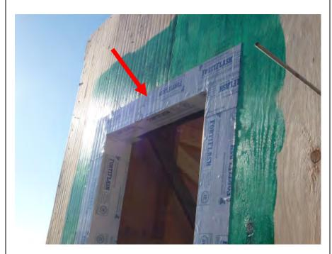
9" wide SAF installed over window head and extended to outside edge of jamb SAF.
