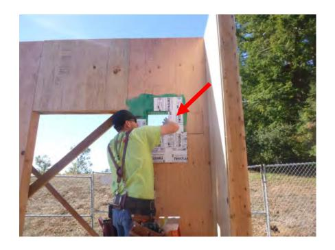
Install SAF along jambs and wrapped into jambs of wall cap R.O.
