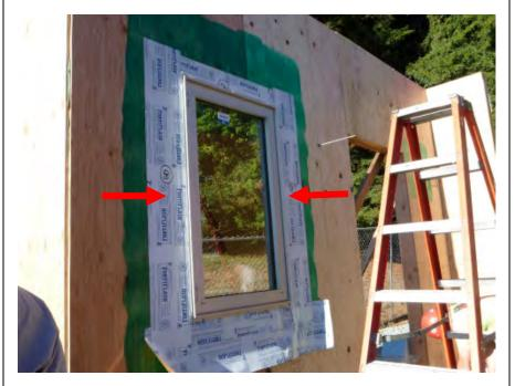
9" wide SAF installed over window flange jambs, extended 6" beyond sill & head rough openings
