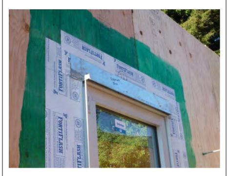
GSM head flashing installed over window head. Fasten using "hot-dip galvanized ring-shank nails". Do not penetrate window head fin with fasteners.
