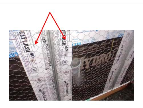
Install SAF in vertical control joint locations over WRB.
