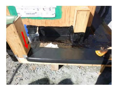
Deck edge uncured neoprene turned up base of column underneath kerf cut.
