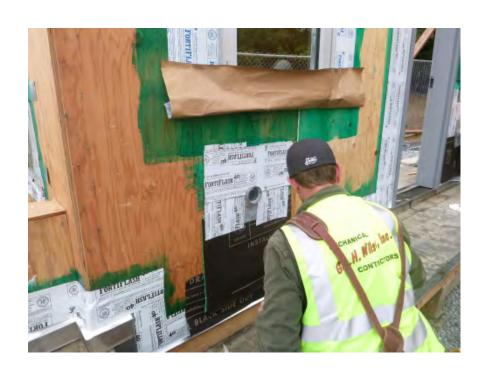
Apply SAF along top flange of electrical box flashing.
