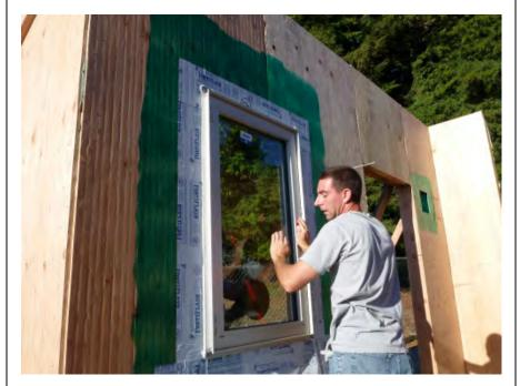
Window installed into rough opening into continuous bead of sealant along head and jambs. Fasten with "S.S. Pan-Head Screws".
