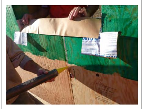
Sealant being applied in sheathing gap greater than 1/8"
