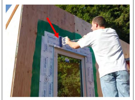
12" wide SAF installed over GSM head flashing.
