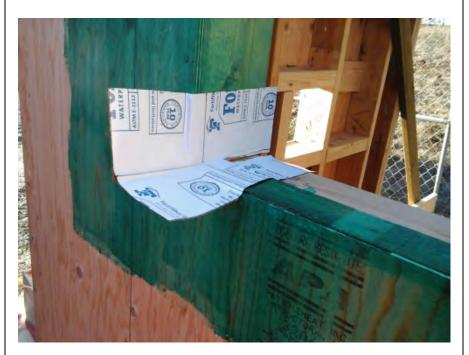
SAF corner pieces installed at bottom corners 4" up jambs.
