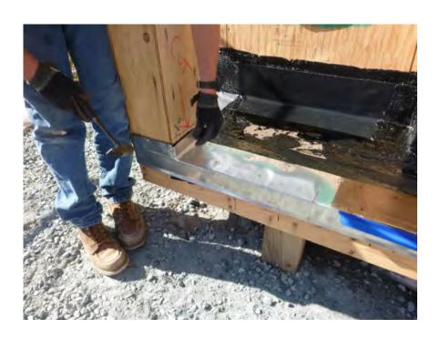
Fully soldered deck edge metal flashing wrapping around deck column. Fasten along top edge of flashing.
