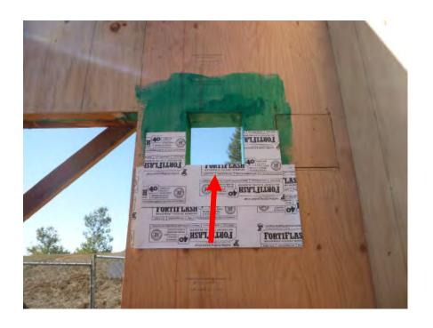
Install SAF along sill and wrapped into sill of wall cap R.O.
