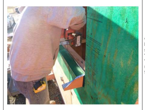
GSM angle with 3/4" vertical leg butted up to tapered shim at sill, secured with "S.S. Pan-Head screws" or "hot-dip galvanized ringshanks nails" into sill framing.
