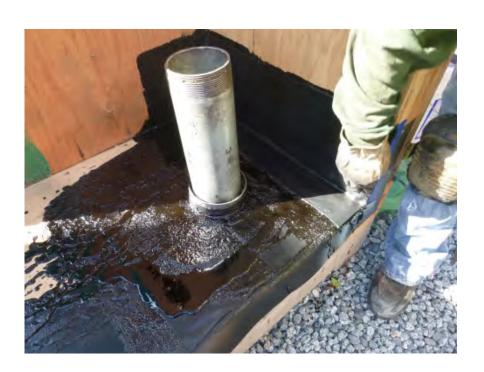
2nd coat of WP membrane applied onto uncured neoprene around pipe collar.
