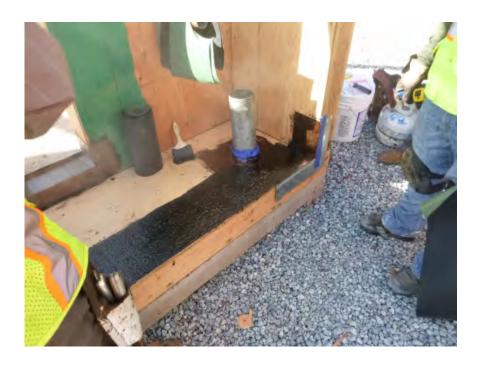
1<sup>st</sup> coat of WP membrane applied onto flange of S.S. pipe collar.
