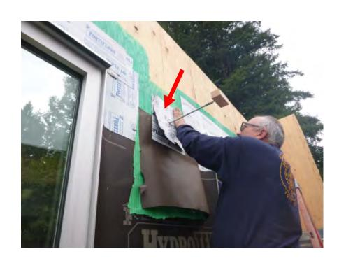
Apply second piece of SAF "head" at bolt, (Step 3)
