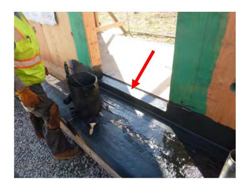
Following the application of 1<sup>st</sup> coat of the WP membrane install the uncured neoprene onto the door sill pan.
