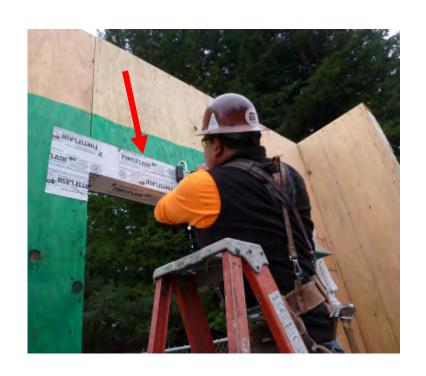
12" wide SAF installed into full depth of rough opening extending out over sheathing 4" min.
