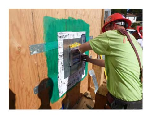
Secure louver to fully soldered collar (see detail). Securing of louver to collar may be done prior to site installation.
