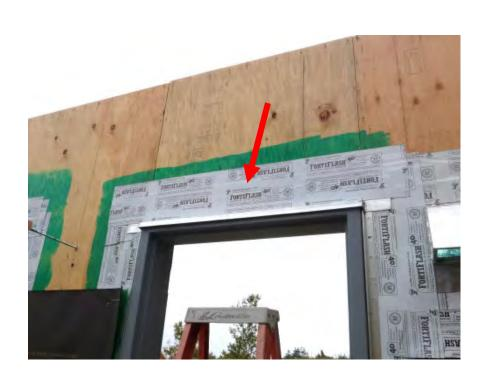
9" wide SAF installed over window head flashing.
