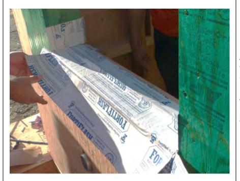
12" wide SAF installed min. 4" over sheathing face, onto the GSM angle to interior edge of sill R.O.
