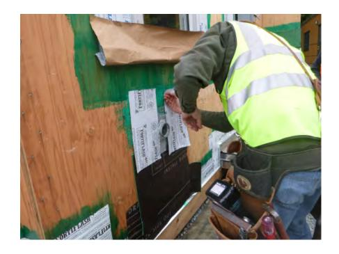
Install 9" wide SAF along jamb flanges of electrical box flashing
