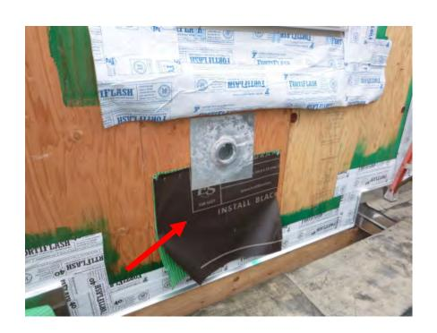
Install starter strip of WRB at sill and secure fully soldered GSM collar around electrical box with "S.S. Pan-Head screws" or "hot-dip galvanized nails" as required.
