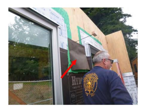
Install starter strip of WRB at sill of tie-bolt to allow for shingling of WRB field installation.
