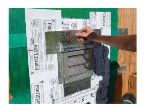
Install GSM head flashing over louver.
