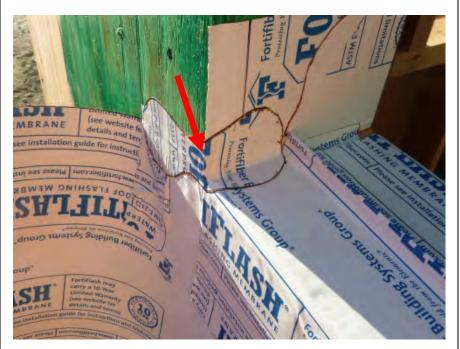
SAF butterflies installed at outside framing corners of sill.
