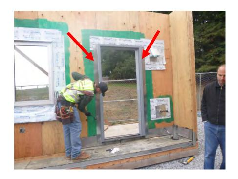
24 GA GSM L-Metal installed, with minimum 1/4" contact between L-Metal and Door Frame, set in sealant.
