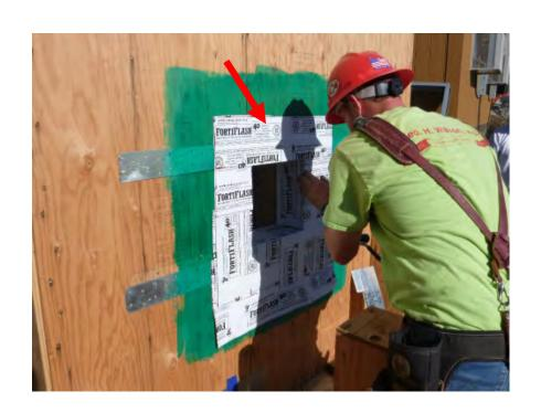
Install SAF along head and wrapped into head of louver R.O.
