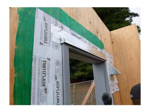
GSM head flashing installed, head flashing to overhang over door frame.
