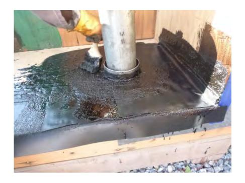
2-pieces of uncured neoprene reinforcement with WP membrane between laps applied around S.S. pipe collar, extending beyond nailing flange onto horizontal deck.
