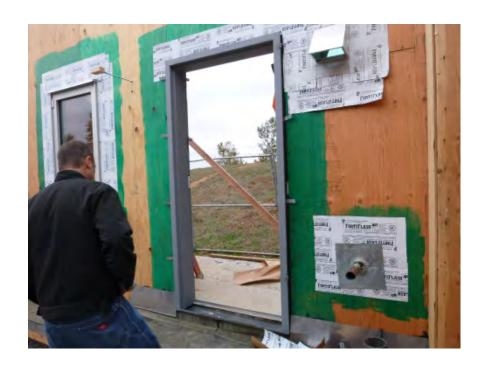
Door frame set into rough opening and secured to structure with "stainless steel pan-head screws" or "hot-dip galvanized ring-shank nails.
