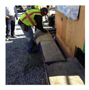
Apply protection course over 2<sup>nd</sup> Coat of podium WP., including onto the sill of door rough opening.
