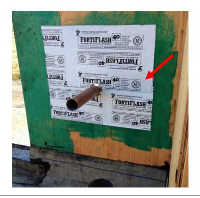
Install SAF along head of pipe penetration, overlapping sill SAF 3" min.
