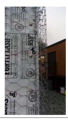
Corner aid installed secured 6" min. o.c.
