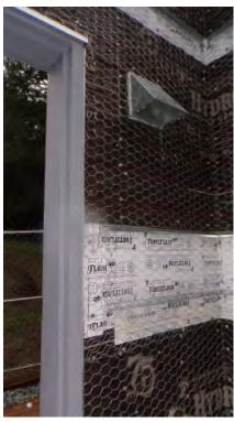
Lath to be secured to structure w/furring nails/screws 16" o.c. horizontally and 6" o.c. vertically.
