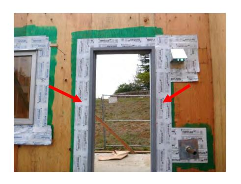
6" wide SAF installed over L-Metal and under plaster stop.
