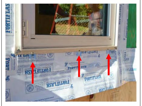
1/16 inch plastic shims installed along sill flange, do not extend past window frame width.
