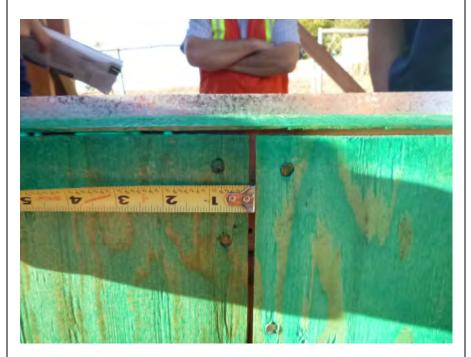
Sheathing to receive SAF with gaps greater than 1/8" to be treated with sealant to provide backing.
