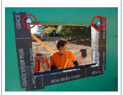
SAF butterfly patches installed at jamb to head framing outside corners.
