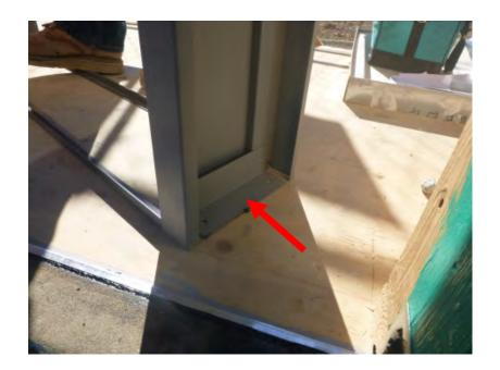
Remove flange from bottom corners of door frame jambs prior to setting into rough opening.
