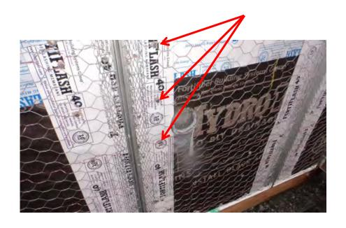
Secure vertical control joint 6" min. o.c
