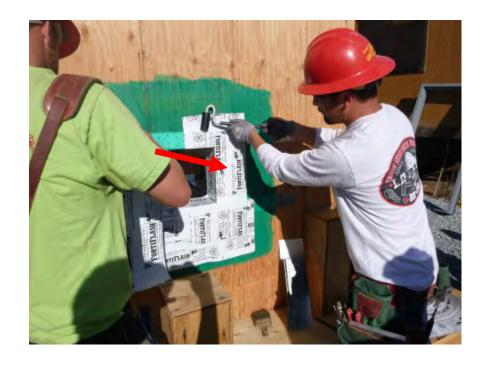
Install SAF along jambs and wrapped into jambs of louver R.O.
