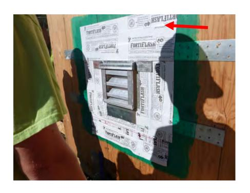
Install SAF over head flashing nailing flange. Pocket where casing bead is covered by head flashing, to be filled with sealant.
