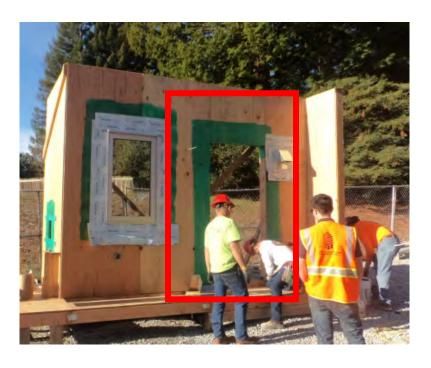
The rough opening is prepared by applying the primer on all sheathing surfaces to receive SAF.
