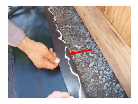
Apply a bonding adhesive (sealant) onto the vertical surface of the deck edge to receive the uncured neoprene
