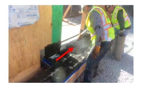
2<sup>nd</sup> Coat of podium waterproofing applied (min. 125 mils) onto reinforcing fabric
