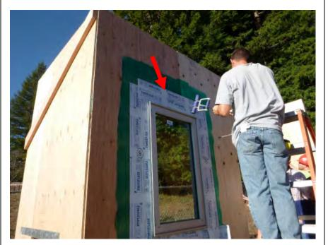
9" wide SAF installed over window head, extended to outside edge of jamb SAF.
