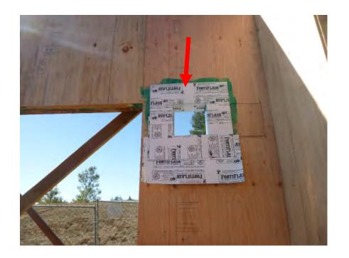
Install SAF along head and wrapped into jambs of wall cap R.O.
