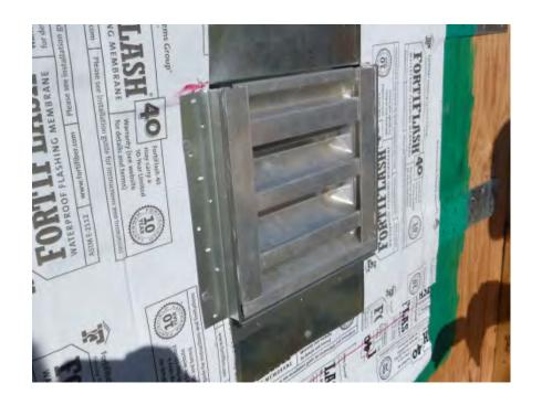
Install casing bead around sill and jambs of louver opening, Apply sealant between louver and casing bead.
