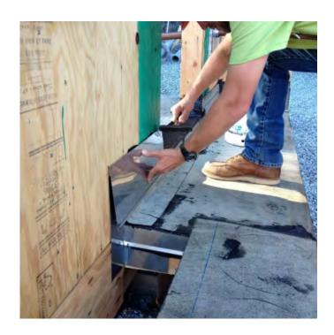
Install UV metal counter flashing with hemmed edge on bottom of leg and fasten with "stainless steel pan-head screws" or "hot-dip galvanized nails".
