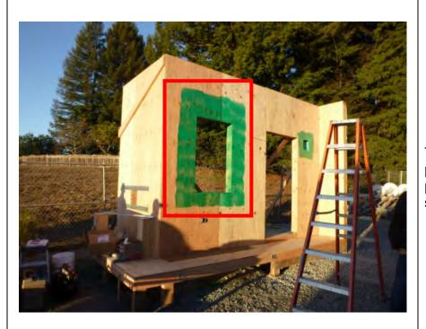
The rough opening is prepared by applying the primer on all sheathing surfaces to receive SAF.
