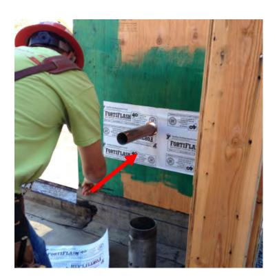
Install SAF along sill of pipe penetration with release paper remaining on bottom half of SAF or provide starter strip of WRB prior to SAF installation.
