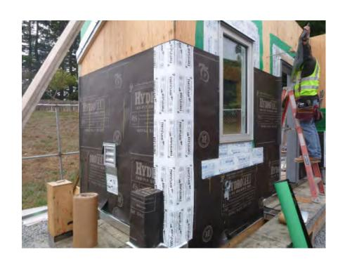
Install WRB in shingled fashion integrating into opening and penetration flashings.
