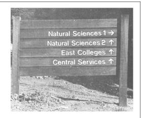
**Current:** Alumalite planks with annodized aluminum H channel with rough-cut 4x4 redwood posts; 2.5" Univers 67 Condensed Bold type.
