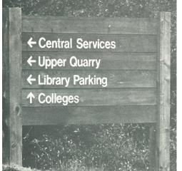
**Current:** Alumalite planks with annodized aluminum H channel with rough-cut 6x6 redwood posts; 4" Univers 67 Condensed Bold type.
