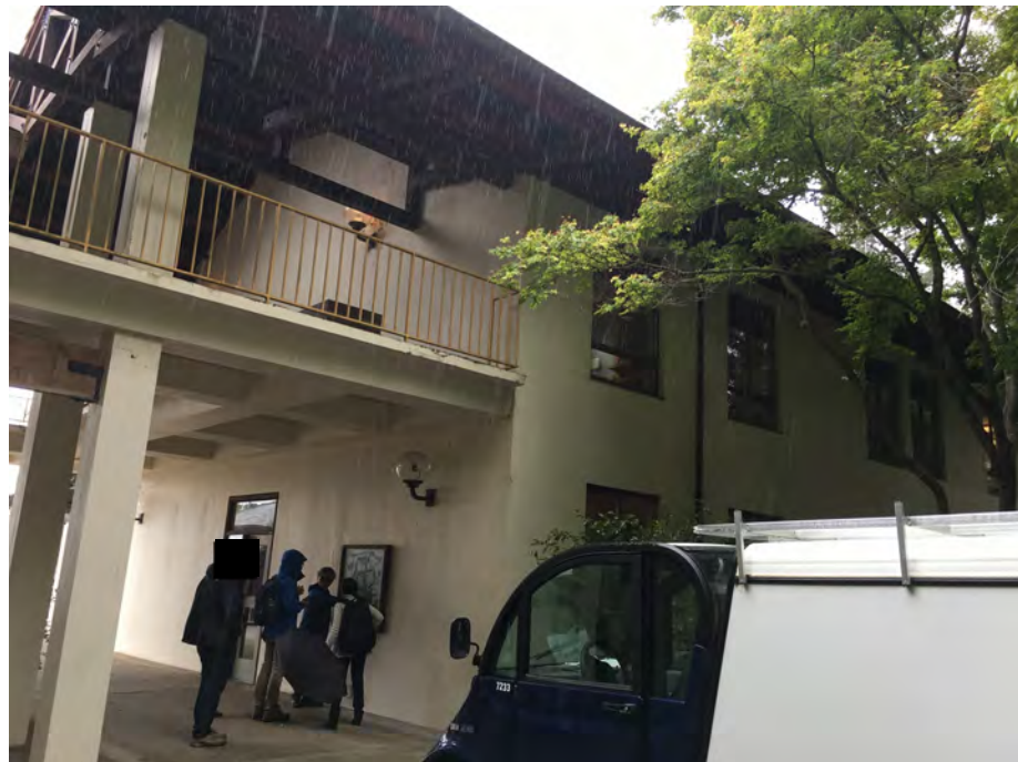
Figure 4 - View of shelter/breezeway to the Academic Building (CAAN 7130)
