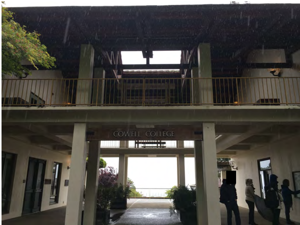
Figure 3 - View of shelter/breezeway from the north side
