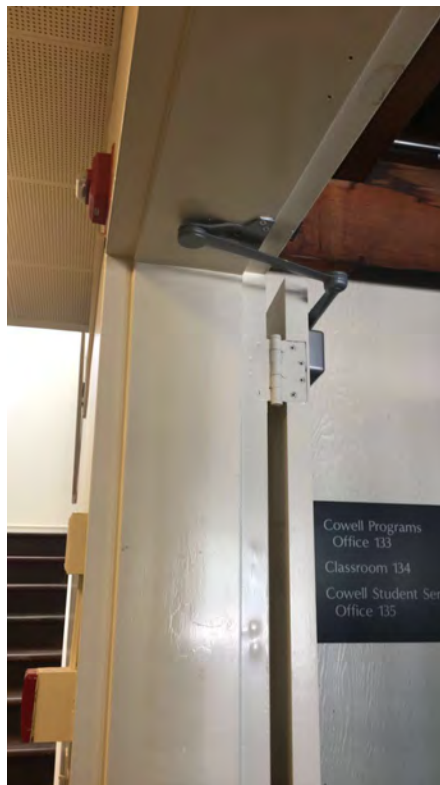
Figure 2 - Door/wall between retrofitted and unretrofitted portion of CAAN 7134 (Cowell College Commons)
