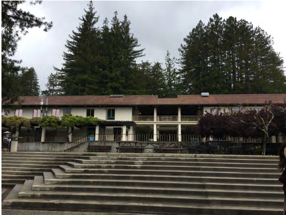
Figure 1 - View from the south with CAAN 7130 (Academic Building) on the left
