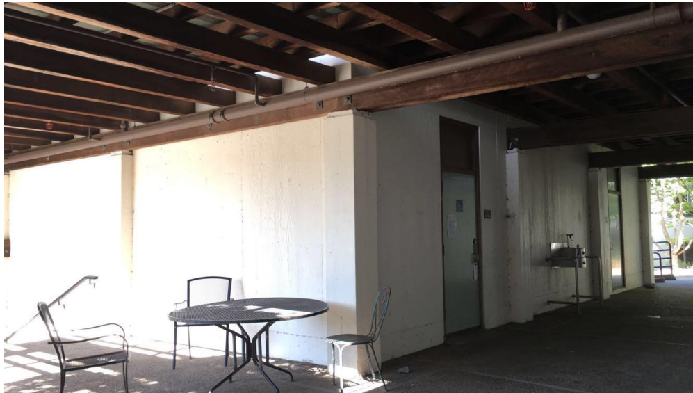
Figure 1 - Doors on northern side of building
