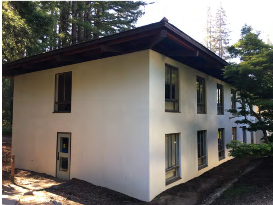
Figure 1 - View from NW corner of the building
