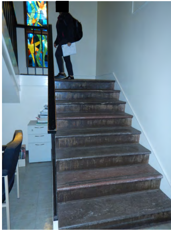
Figure 5 - Stairs at NE corner of the building
