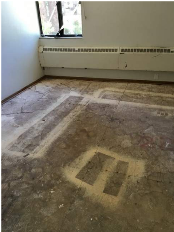
Typical plywood sheathing on building floors
