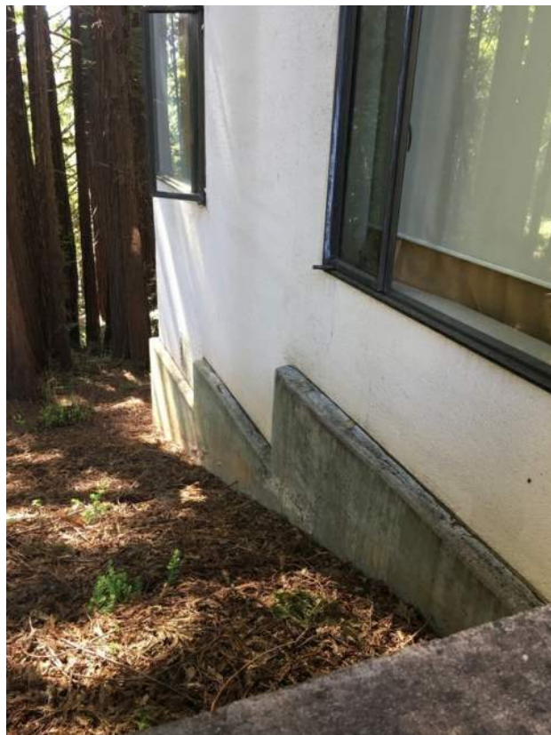
Stepped footing at crawl space
