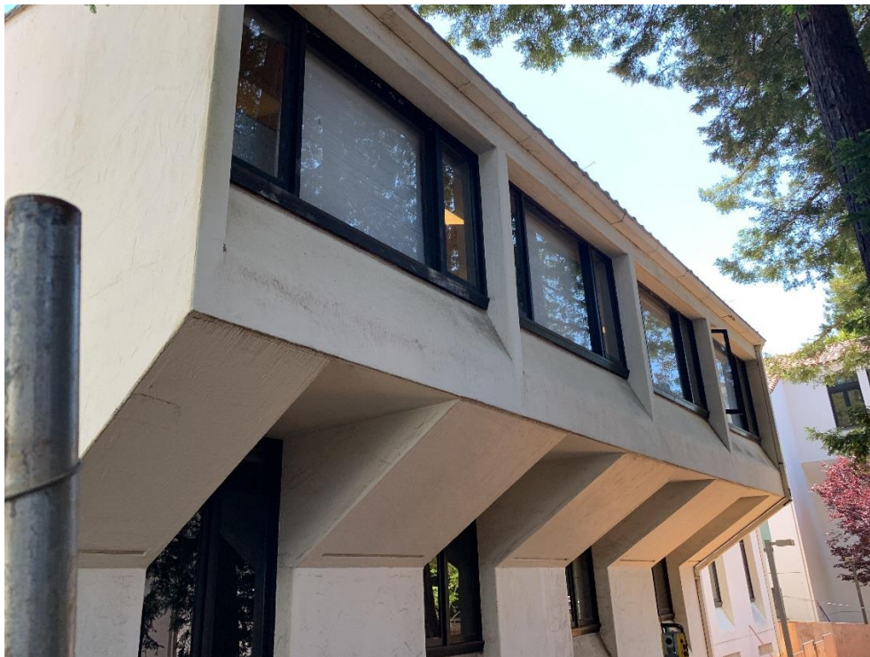
Detail of Overhang at East Elevation (Looking Northwest)
