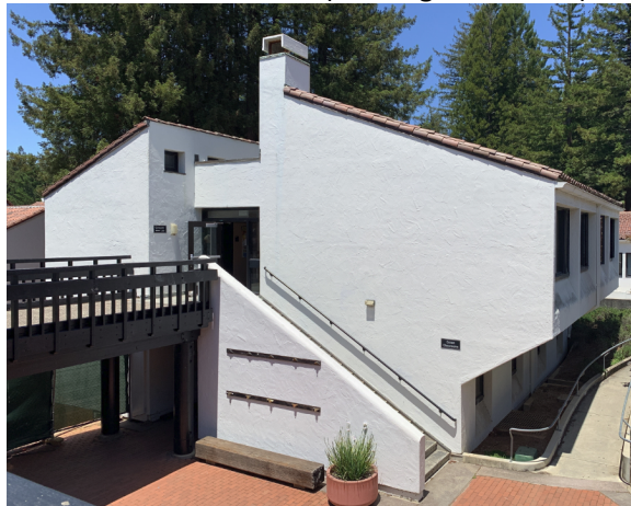
South Elevation (Looking Northwest)
