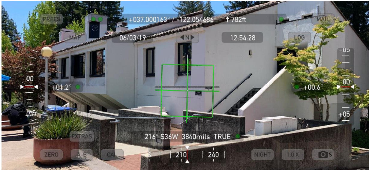
Northeast Corner (Looking Southwest)
