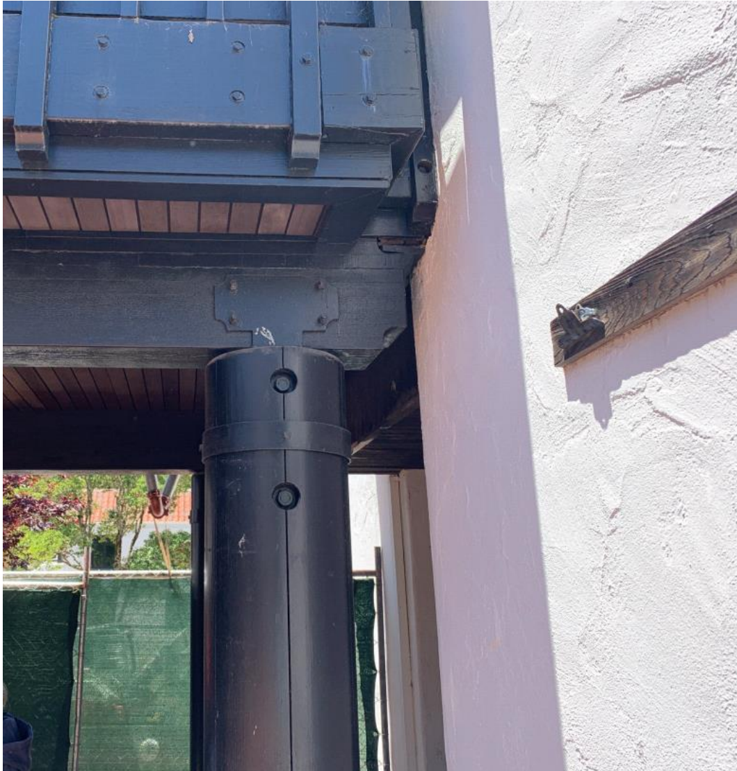
Close-up of Walkway Adjacent to South Elevation
