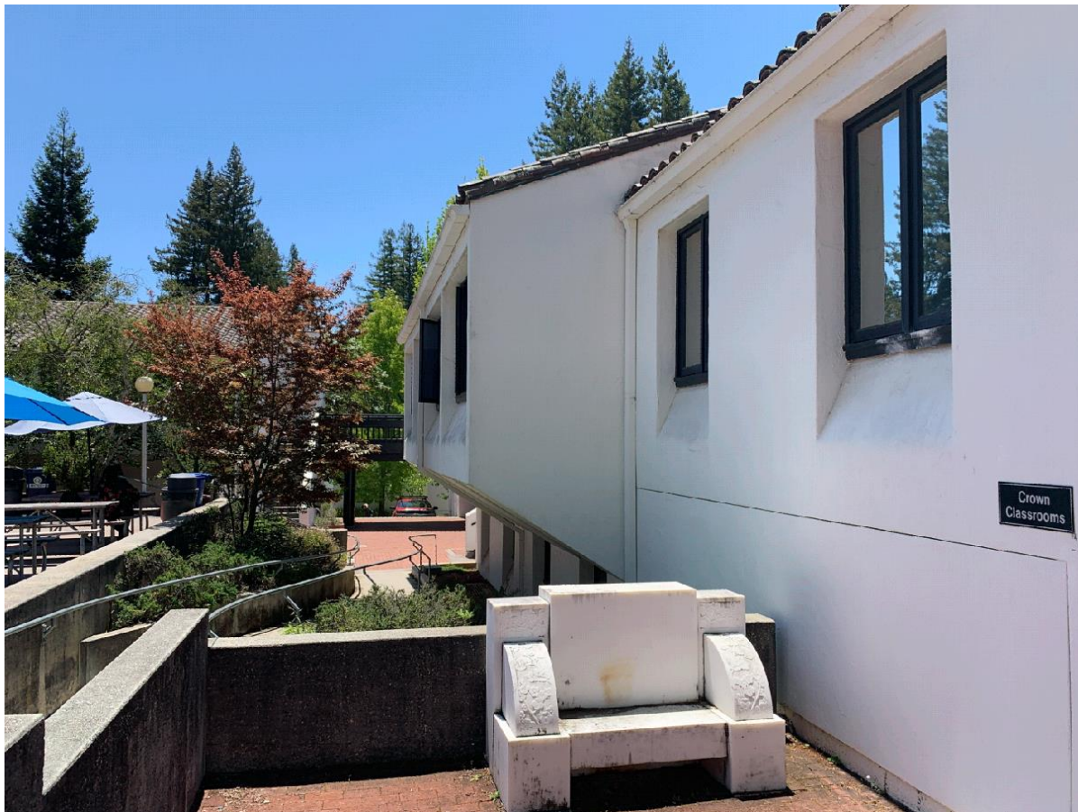
East Elevation (Looking South)
