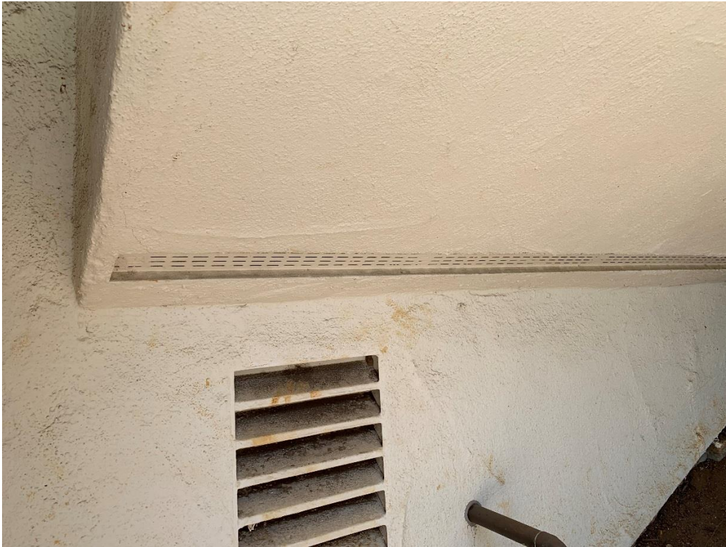
Continuous Vent Below Overhang at South Elevation of 1985 Addition
