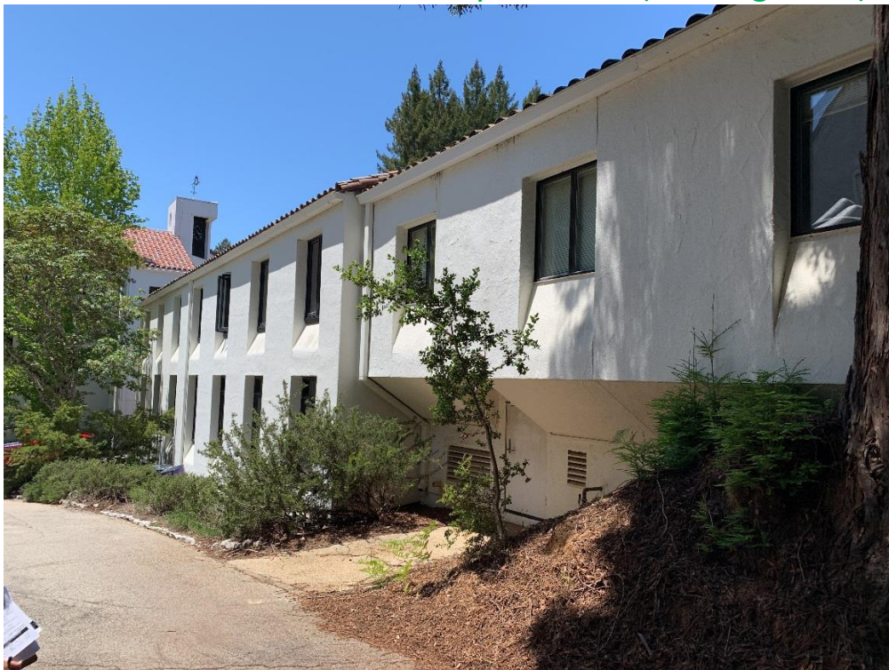
South Elevation (Showing Interface Between 1967 and 1985 Construction)
