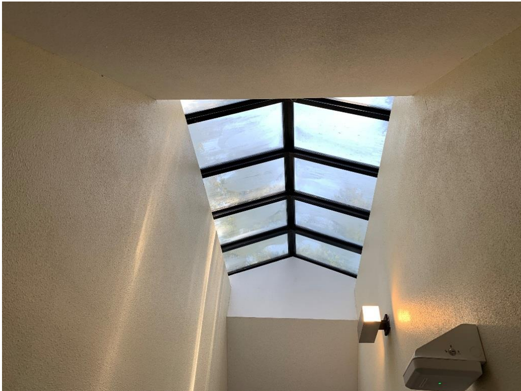
Skylight in Corridor of 1985 Addition
