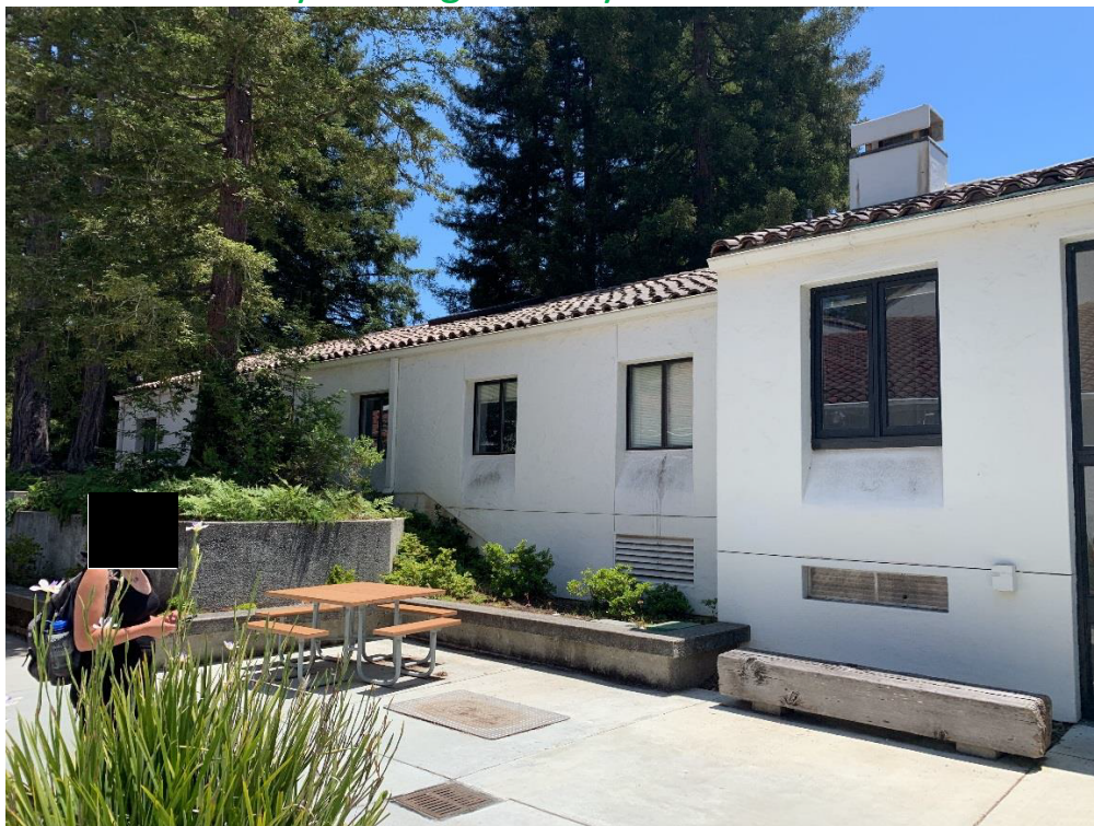
Partial North Elevation, Two-Story Portion in Foreground, One-Story Addition in Background
