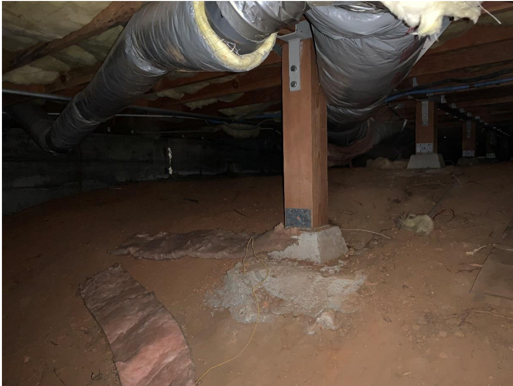
Interior Posts Viewed from Partial Basement of 1985 Addition
