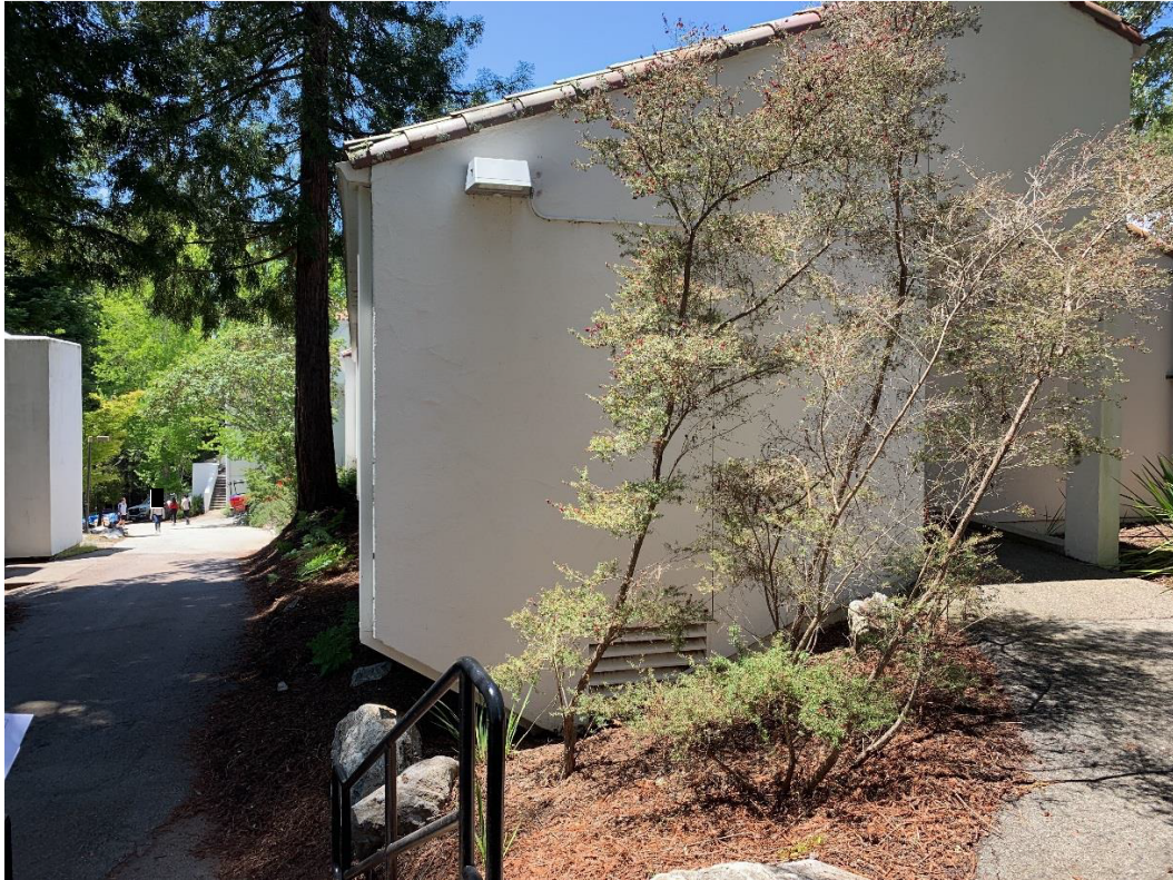
East Elevation 1985 One-Story Addition (Looking West)
