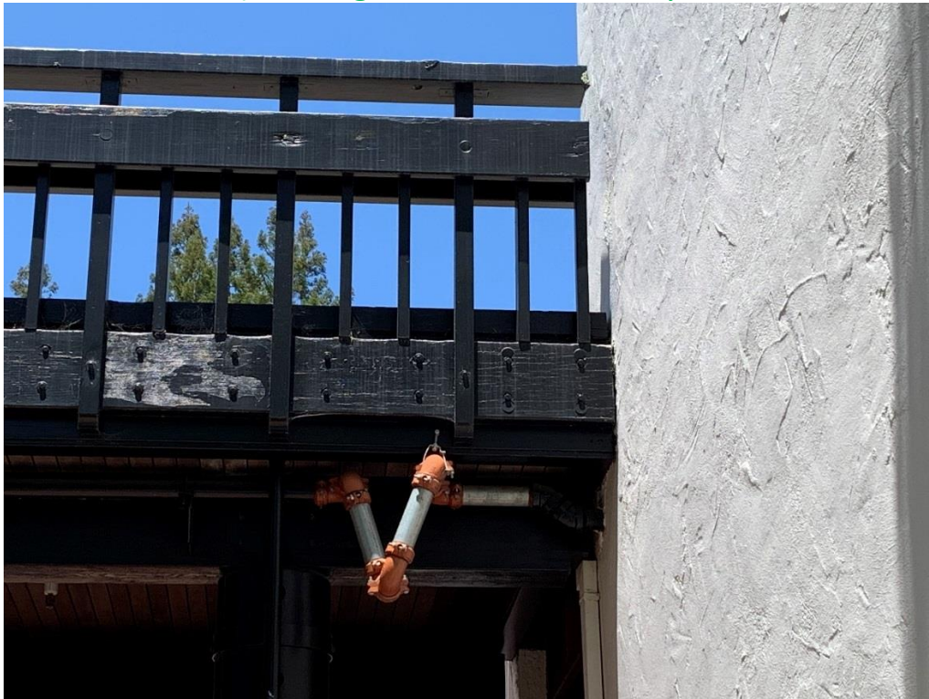
Close-up of Walkway Adjacent to West Elevation
