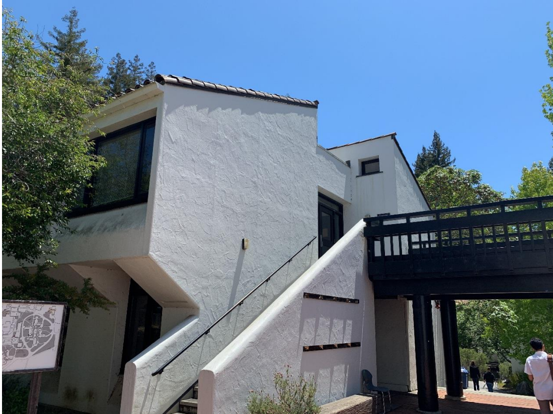
West Elevation Original 1967 2-Story Faculty Wing (Looking Southeast)
