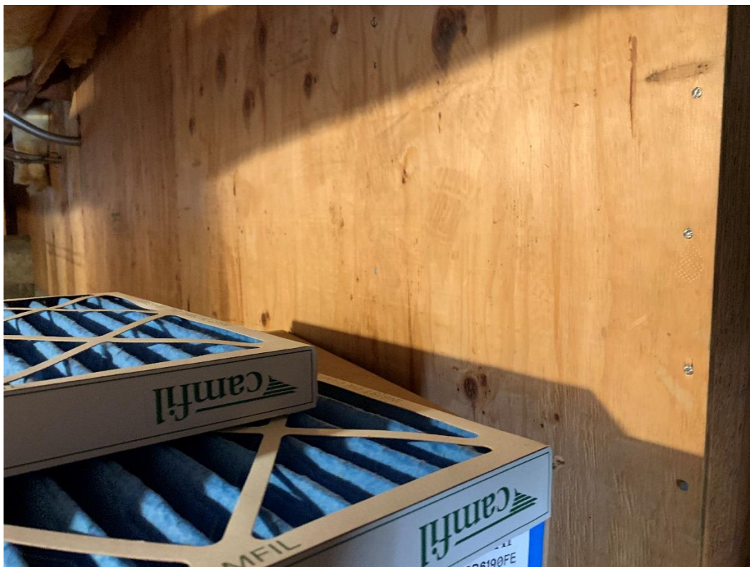
Transverse Shear Wall in Partial Basement of 1985 Addition
