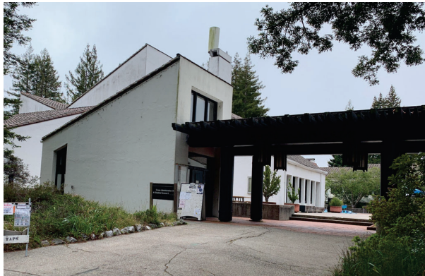
North facade and pergola (looking southeast)
