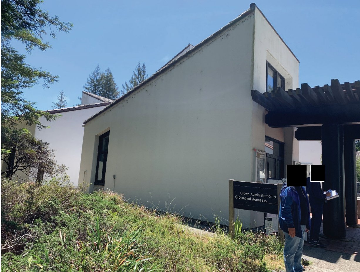
Northwest Corner of Gatehouse (Looking Southeast)
