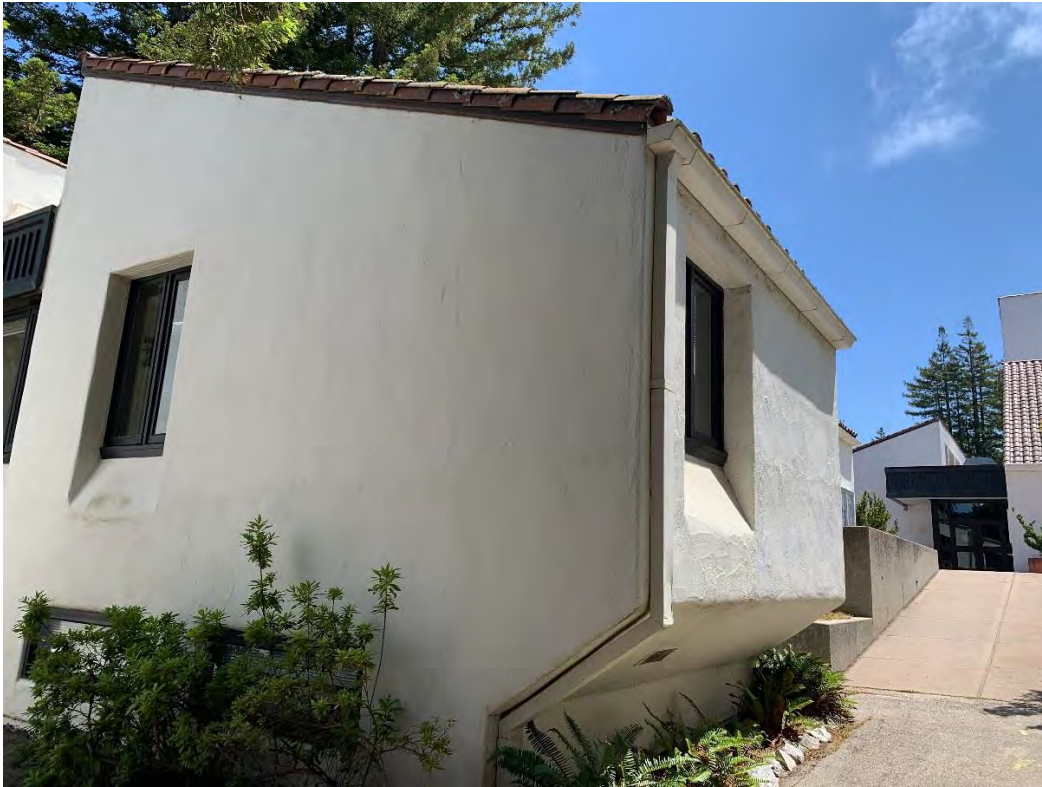
Southwest Corner with Overhang (Looking Northeast)
