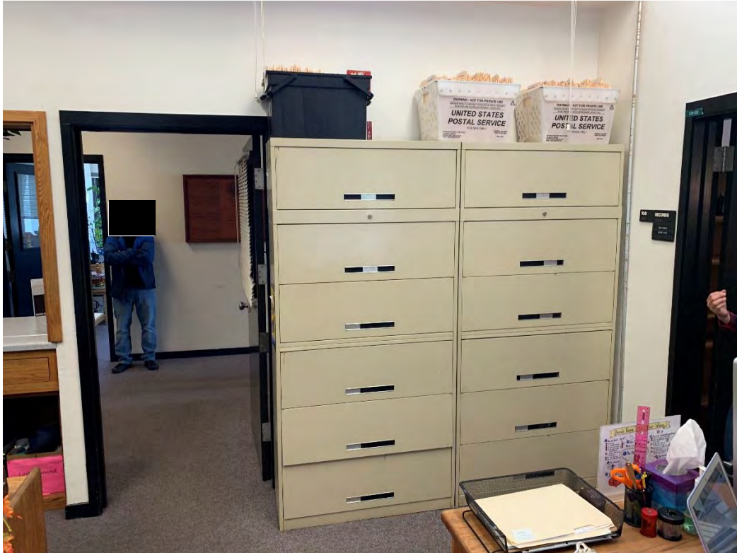
One Wall Anchor Visible at Tall Cabinet
