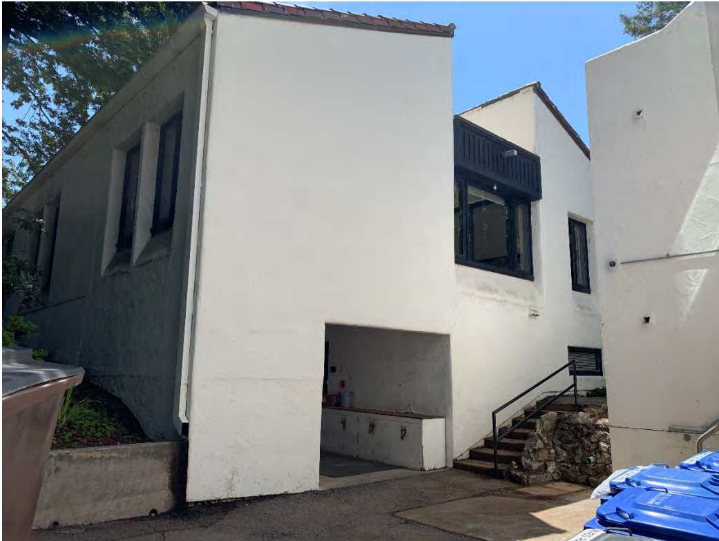
Northwest Corner at Entry to Basement Area (Looking Southeast)
