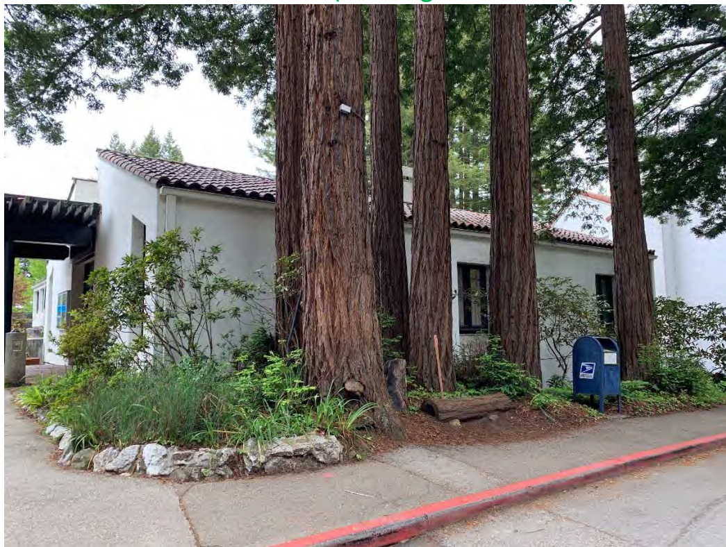
North Elevation (Looking Southwest)
