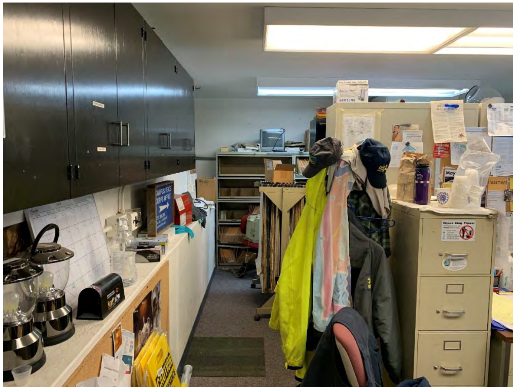
Unanchored File Cabinets and Tall Shelving in Basement Office
