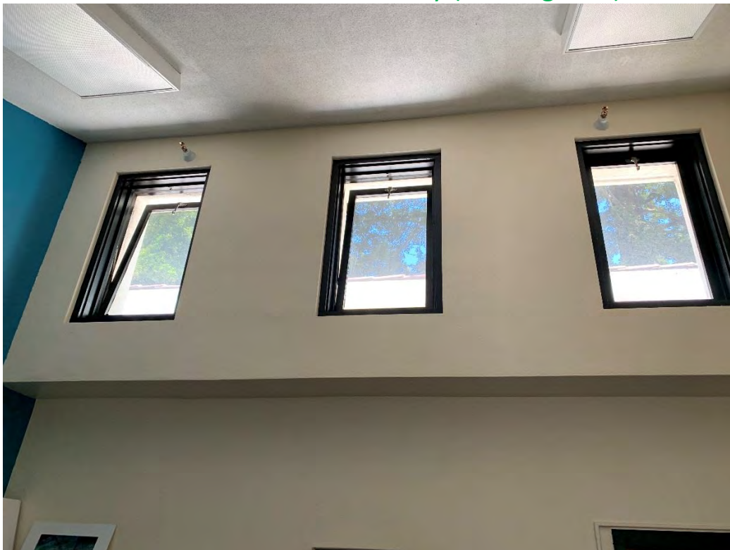
Clerestory Windows above Corridor Walls (Looking North)
