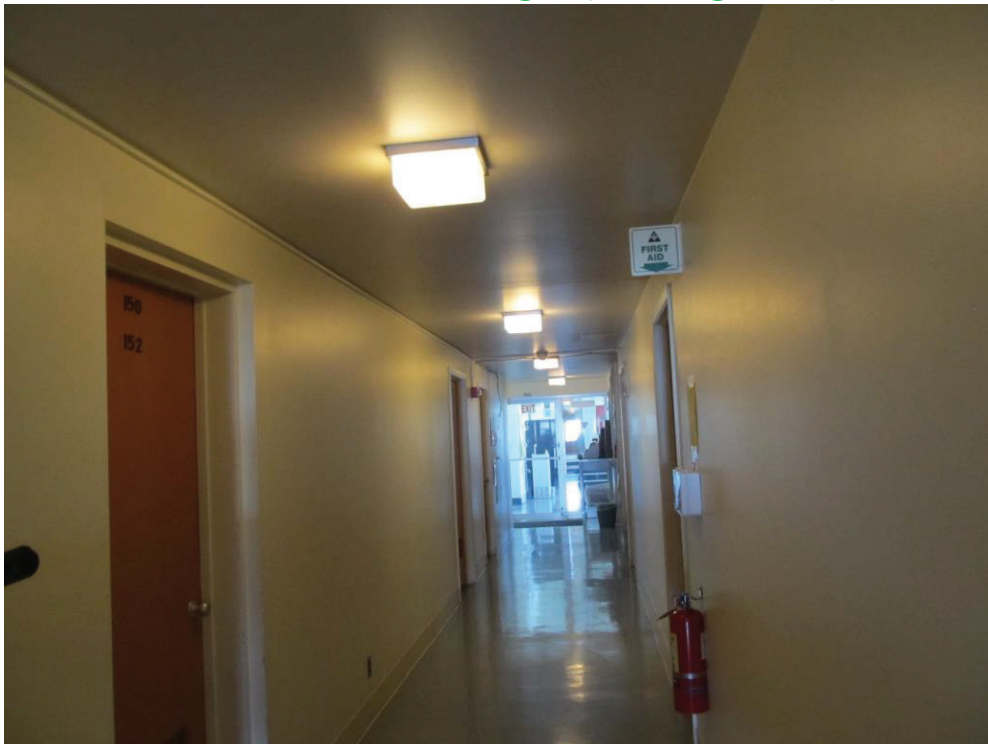
Typical Interior Corridor
