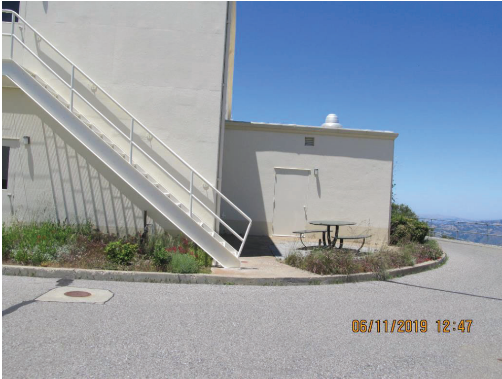
East Elevation (Two-Story Portion at Left, One-Story Portion at Right, Looking West)
