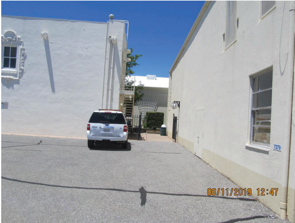
South Elevation at Right (Looking West)
