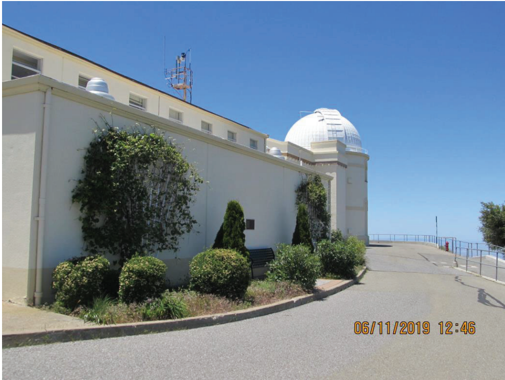
North Elevation of One-Story Portion (Looking West)
