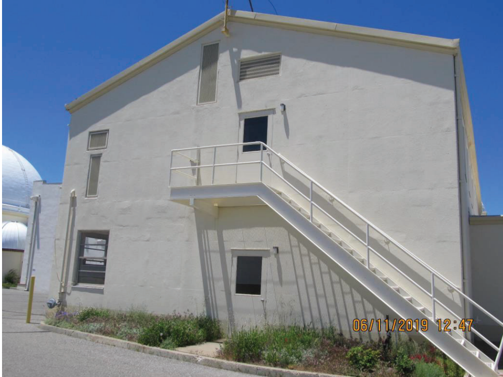
East Elevation (CIP Gable Wall, Looking West)
