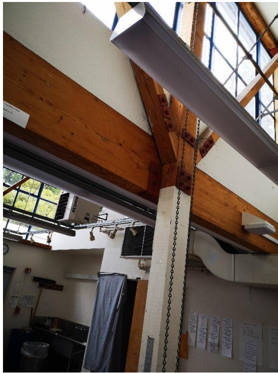
Close-up of Brace-to-Column Details (Detail C/S6)
