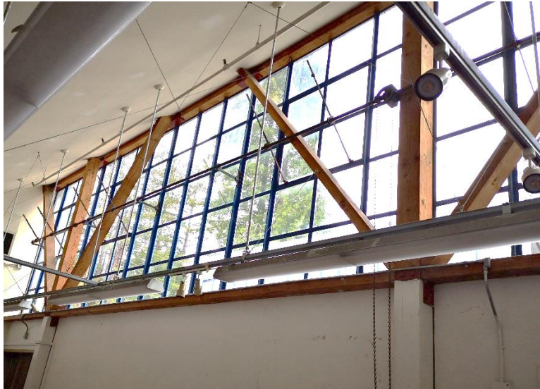
Wood Braced Frame at Exterior Wall
