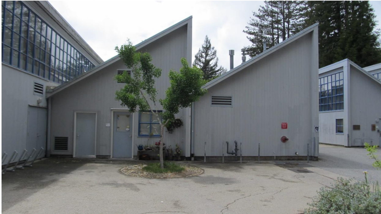
Partial East Elevation (Looking East from Middle Courtyard)
