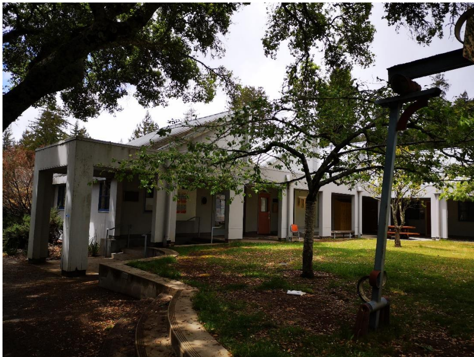
Southeast Corner (Looking Southwest from South Courtyard)
