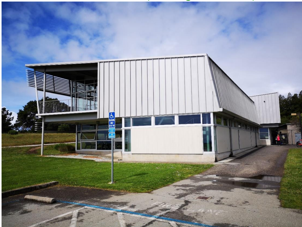
Northeast Corner (Looking Northwest)
