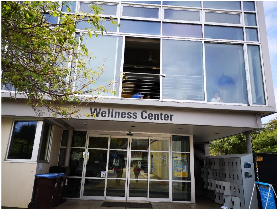
Entrance (North Elevation Looking South)
