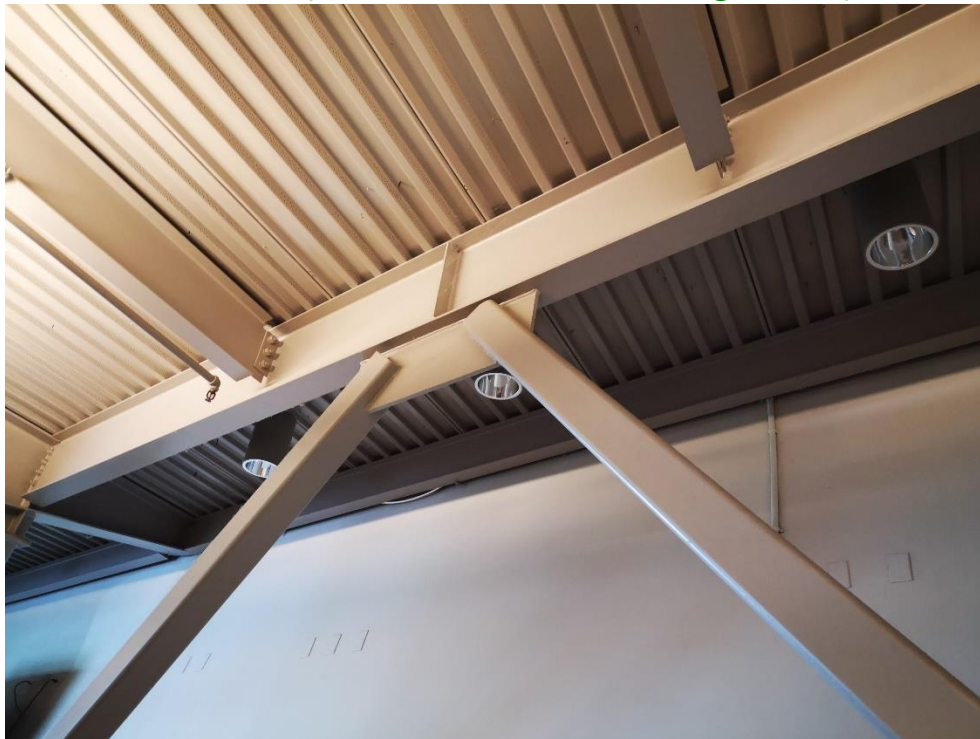
Brace Elements and Metal Deck Roof
