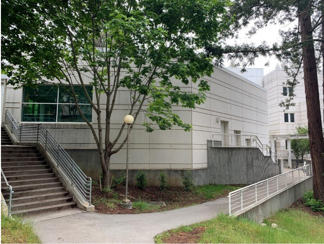
Southwest Elevation Building B
