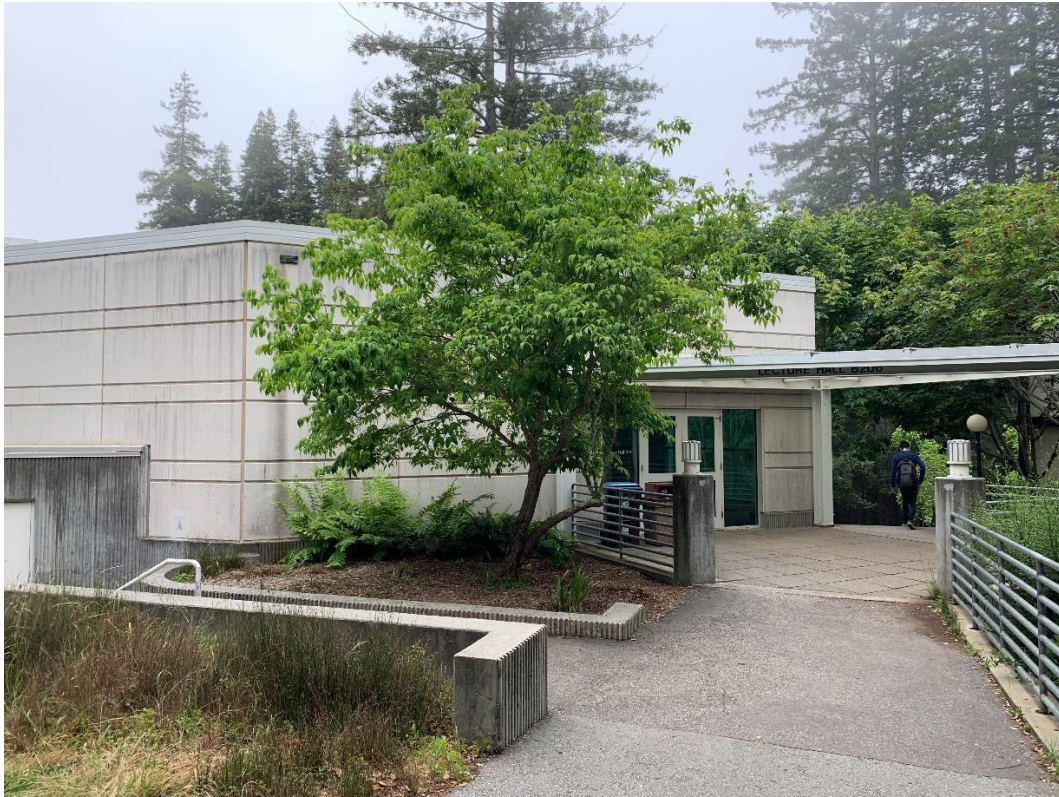
Lecture Hall B206 Entry at North Elevation (Looking Southwest)
