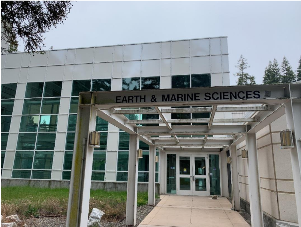
Atrium North Elevation and East Wall of Lecture Hall B206 at Right (Lecture Hall Exit via Atrium)
