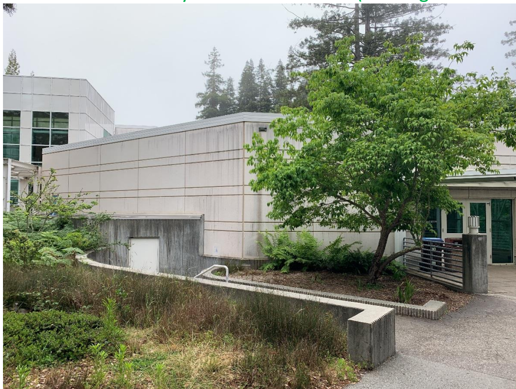
Lecture Hall (Looking Southwest, Atrium at Left)
