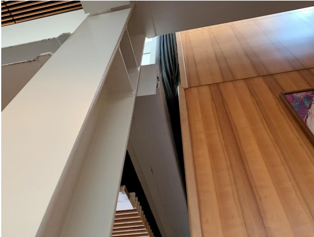
Interior View Looking Up at Boundary Between Building B and Atrium
