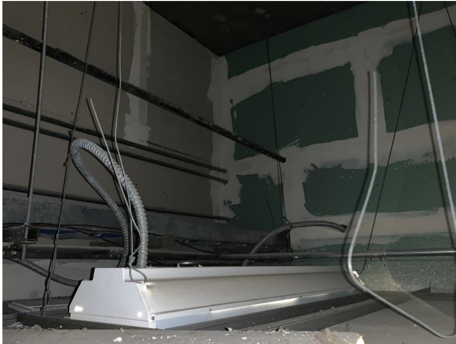
Building C (Typical View Above Ceiling)
