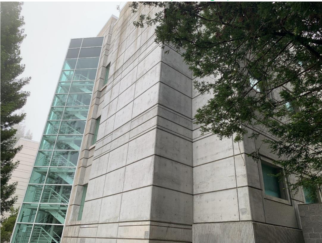
Southeast Corner (Building D)
