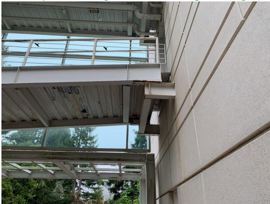
Bridge Support Detail (Looking South, Building A1 at Right)
