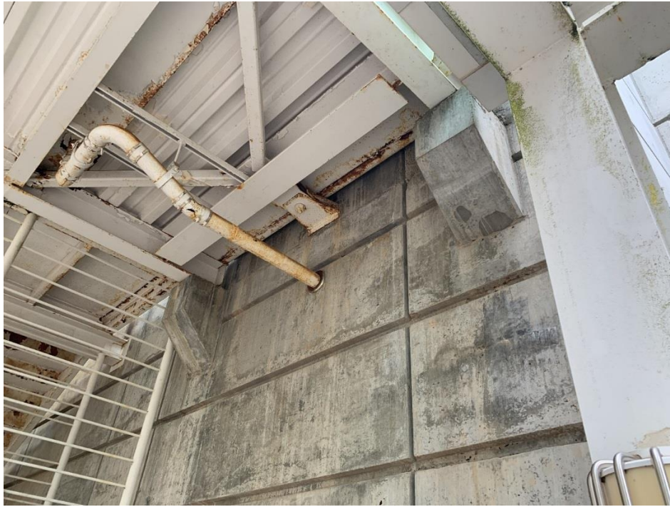
Bridge Support Detail (Looking North, Anchored to Building D at Right)
