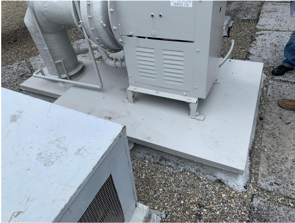
Anchored Equipment at Roof (Building D)
