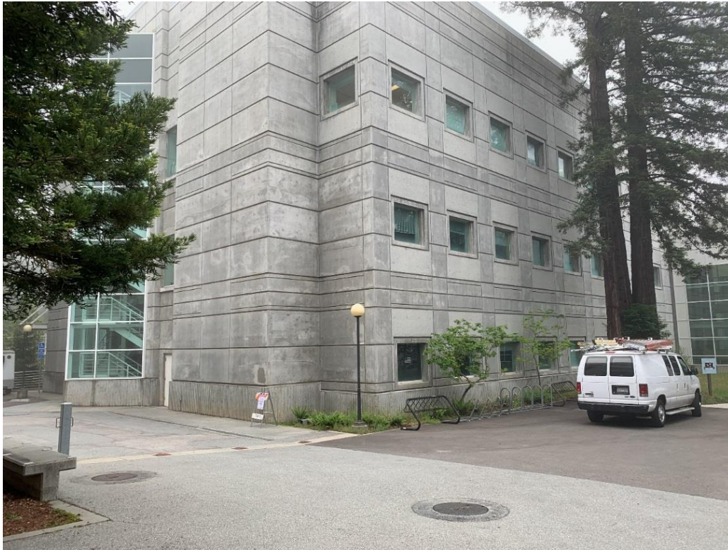
Building C (Northwest Corner)
