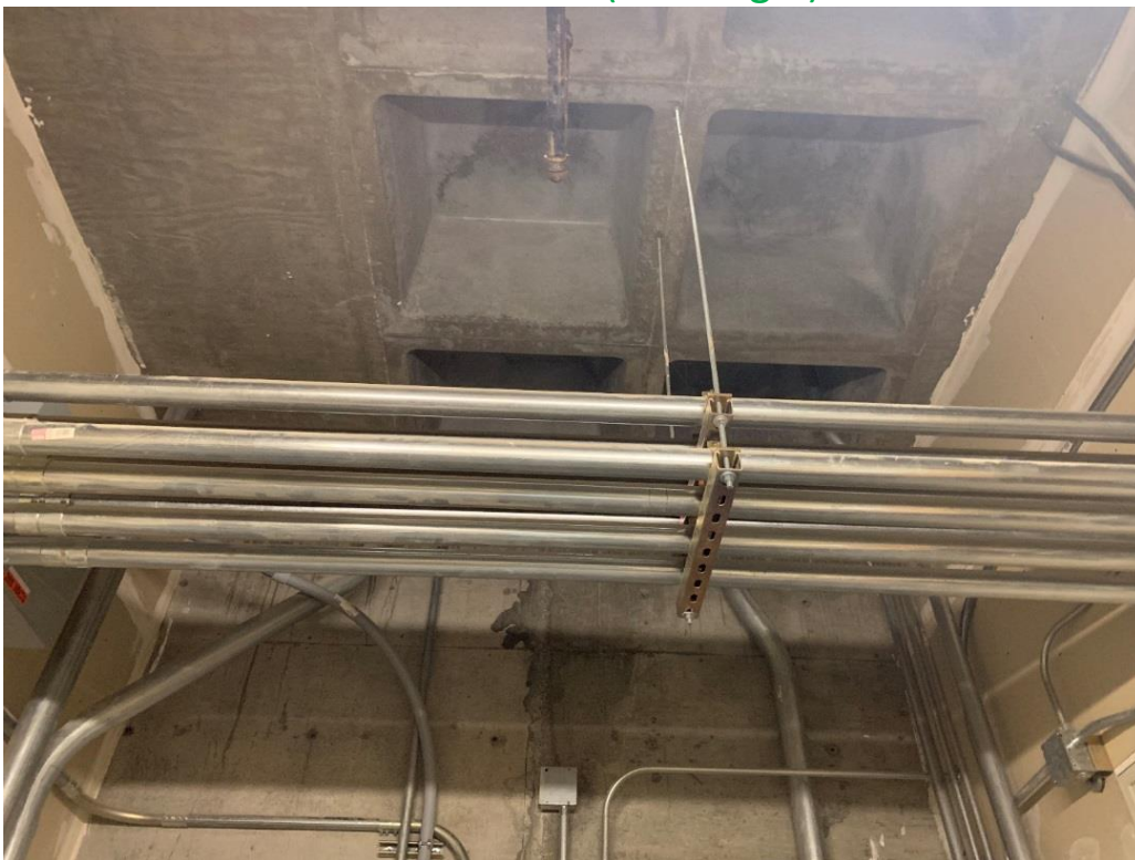
Building C (View Above Ceiling in Corridor near C300)
