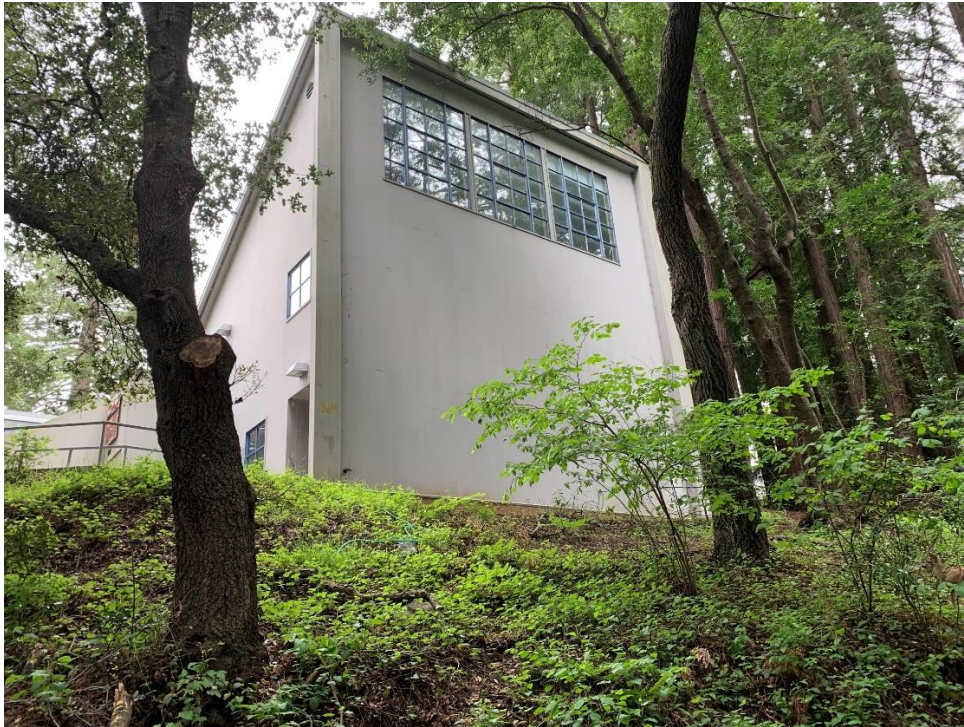
Reference north wall with large window
