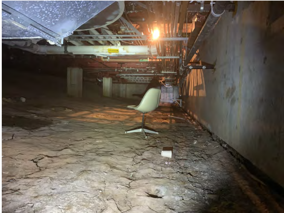
Foundation crawl space
