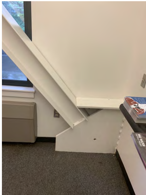
Coped flange at brace gusset
