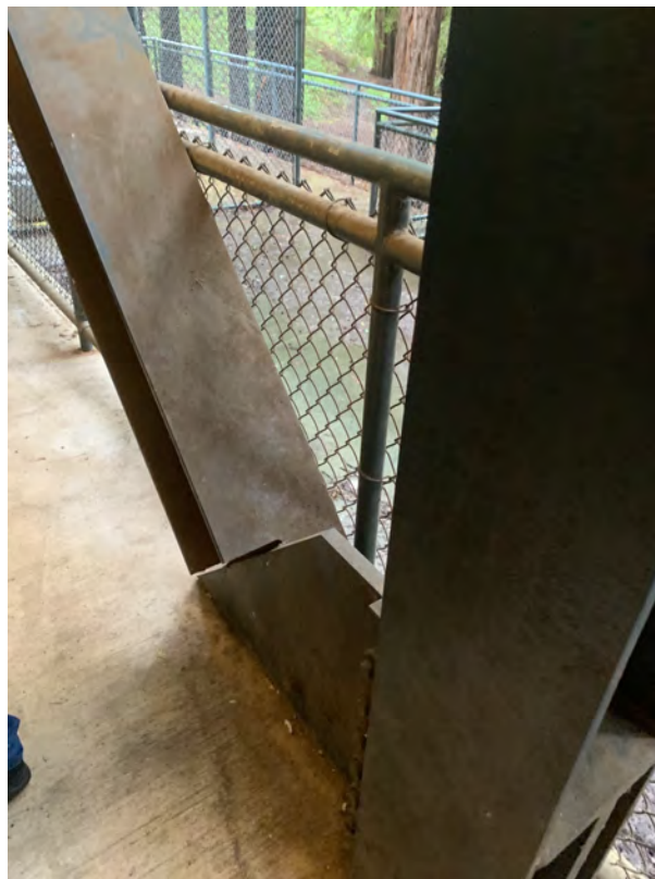
Lower Ground Floor - Coped flange at brace gusset
