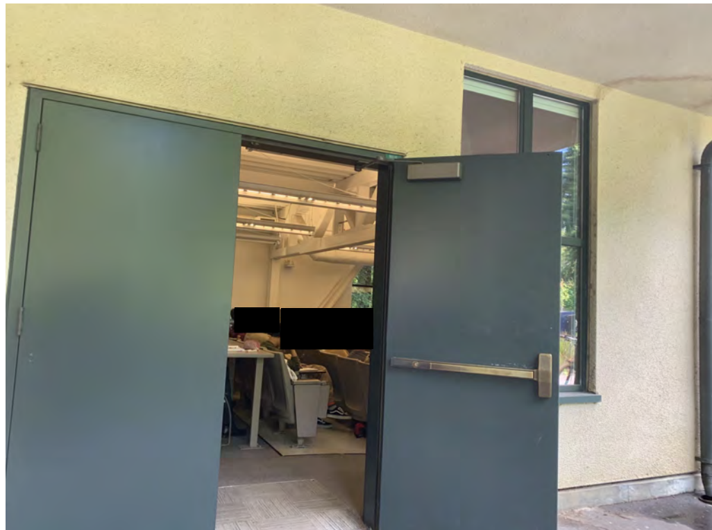
Transfer truss in lecture hall
