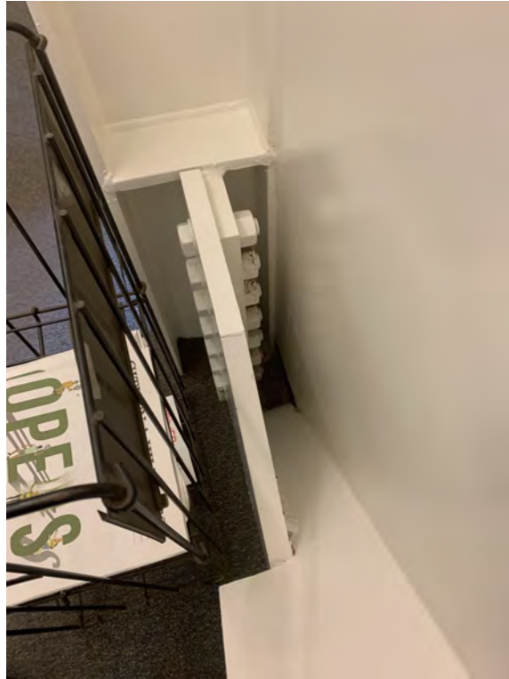
Coped beam flange
