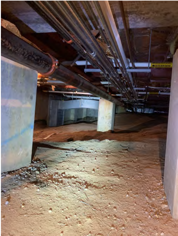
Foundation crawl space
