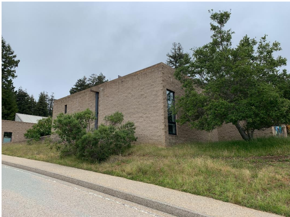
Southwest corner (Looking northeast)
