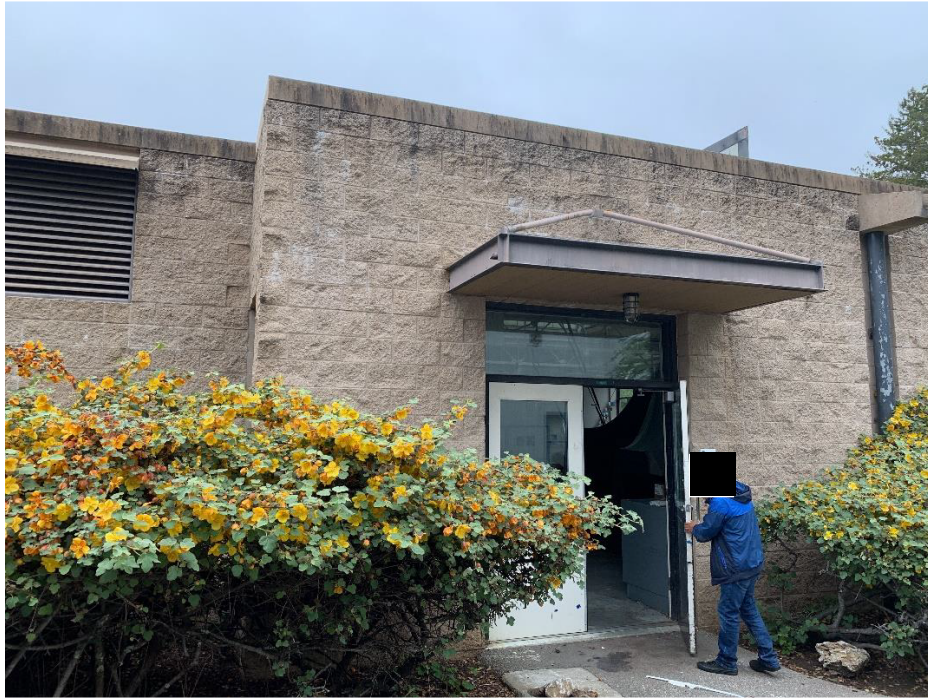
Partial east elevation (looking east)
