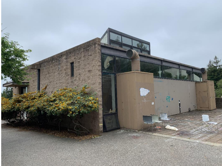
Northeast corner (Looking southwest)
