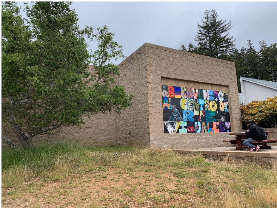
Partial south elevation (looking northwest from the street)
