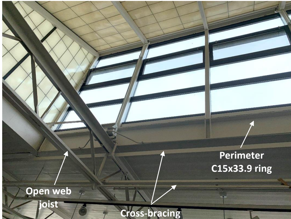
Skylight (looking southeast)
