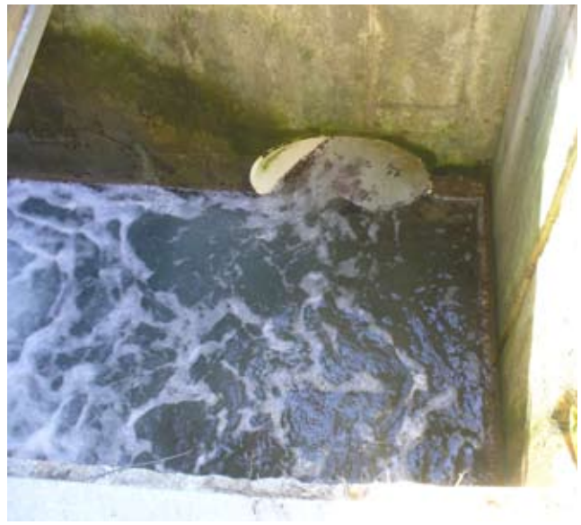
Lower Terrace seawater outfall vault
