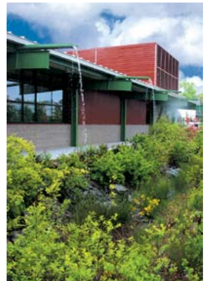
Examples of 'LID' measures; a roof downspout and water quality planter (right) and a parking lot featuring pervious pavement (below.)
