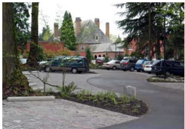
Examples of 'LID' measures; a roof downspout and water quality planter (right) and a parking lot featuring pervious pavement (below.)
