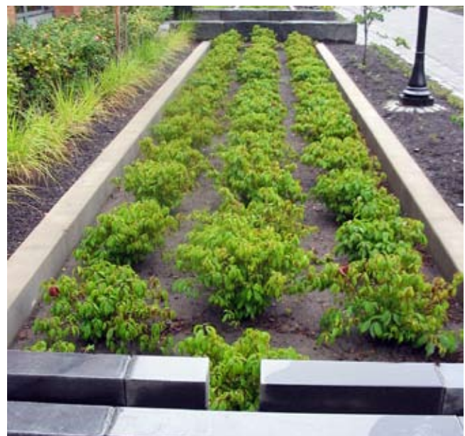
Stormwater filtration planter, Lewis and Clark College, Portland, Oregon
