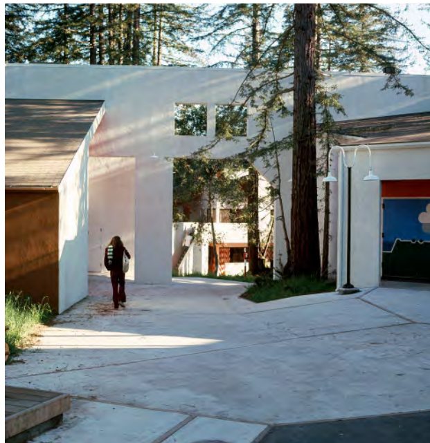
Fig. 4.1.3-2 Accent color on face of add-on elements (Left: G2/A2 Historic Archway, Right: R8) (Kresge College, Morely Baer Photographs - UCSC) Archives)
