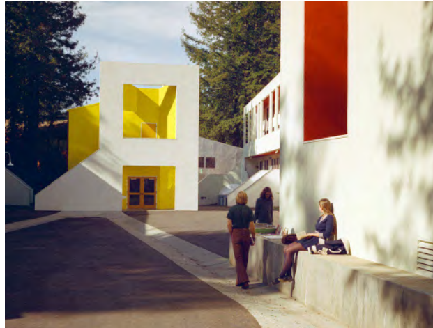
Fig. 4.1.3-2 Accent color on interior faces of trivial monuments (Left: A1, Right: A2) (Kresge College, Morely Baer Photographs - UCSC)
