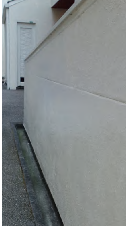
Fig. 3.2.5-1 Existing stucco finish and panel reveal (R1)
