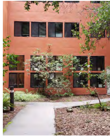
Fig. 4.1.2-1 Rust color used at secondary facades (R12, R13) (Kresge College, Morely Baer Photographs - UCSC) Archives)
