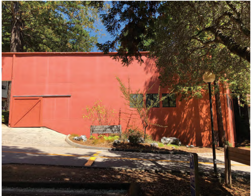
Fig. 2.2-20 Woods-facing facade with darker color and barn door
