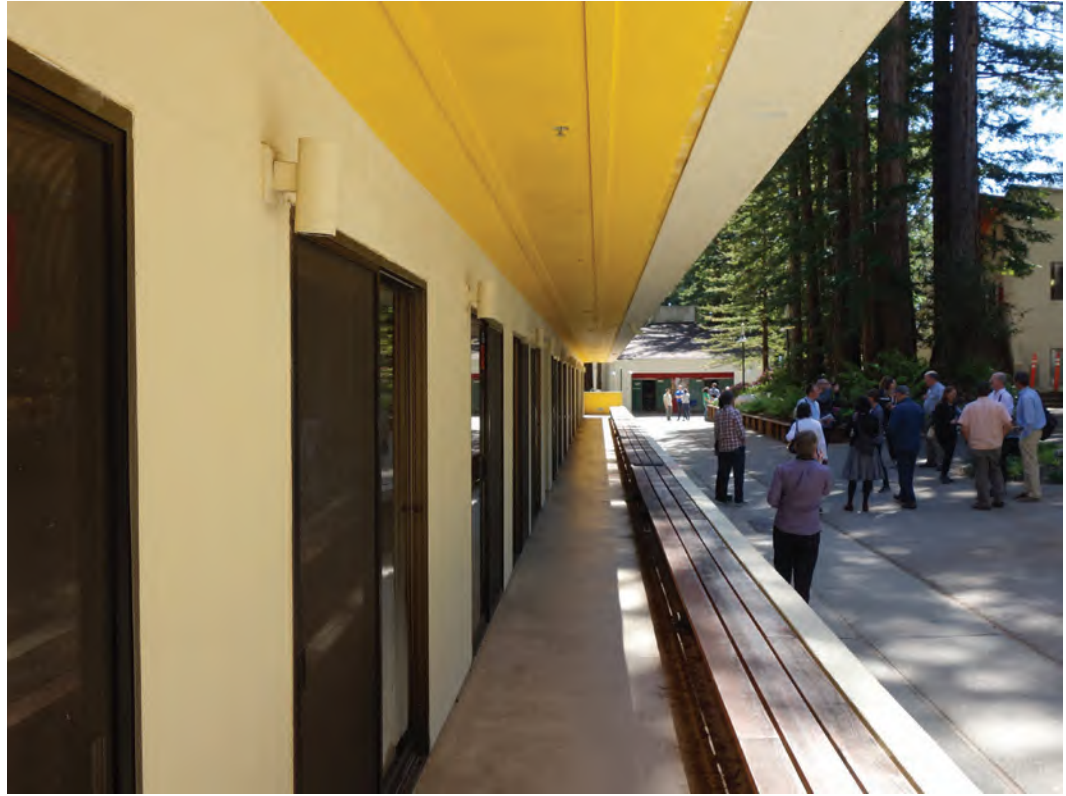
Fig. 3.2.6-11 Existing bench flush with pony wall (R8)
