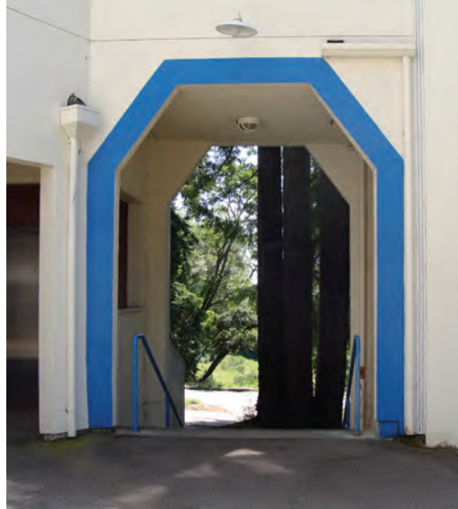
Fig. 2.2-23 Supergraphic and accent railings at opening between R12 and A1
