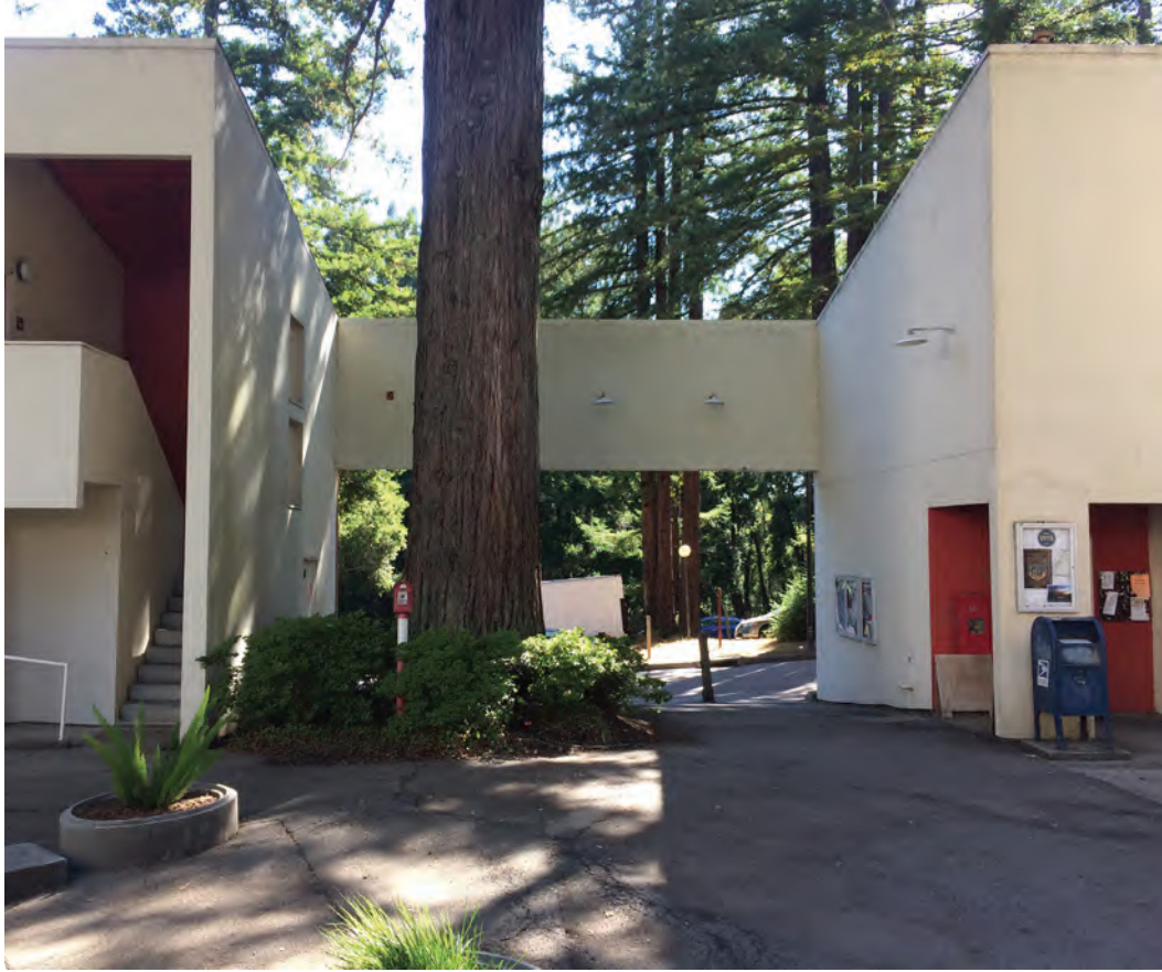
Fig. 2.2-21 Piazzetta / street- facing facade and connection to R13
