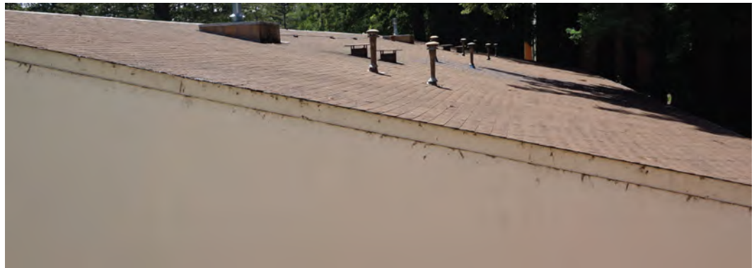
Fig. 3.2.5-7 Existing roof eaves (R1)
