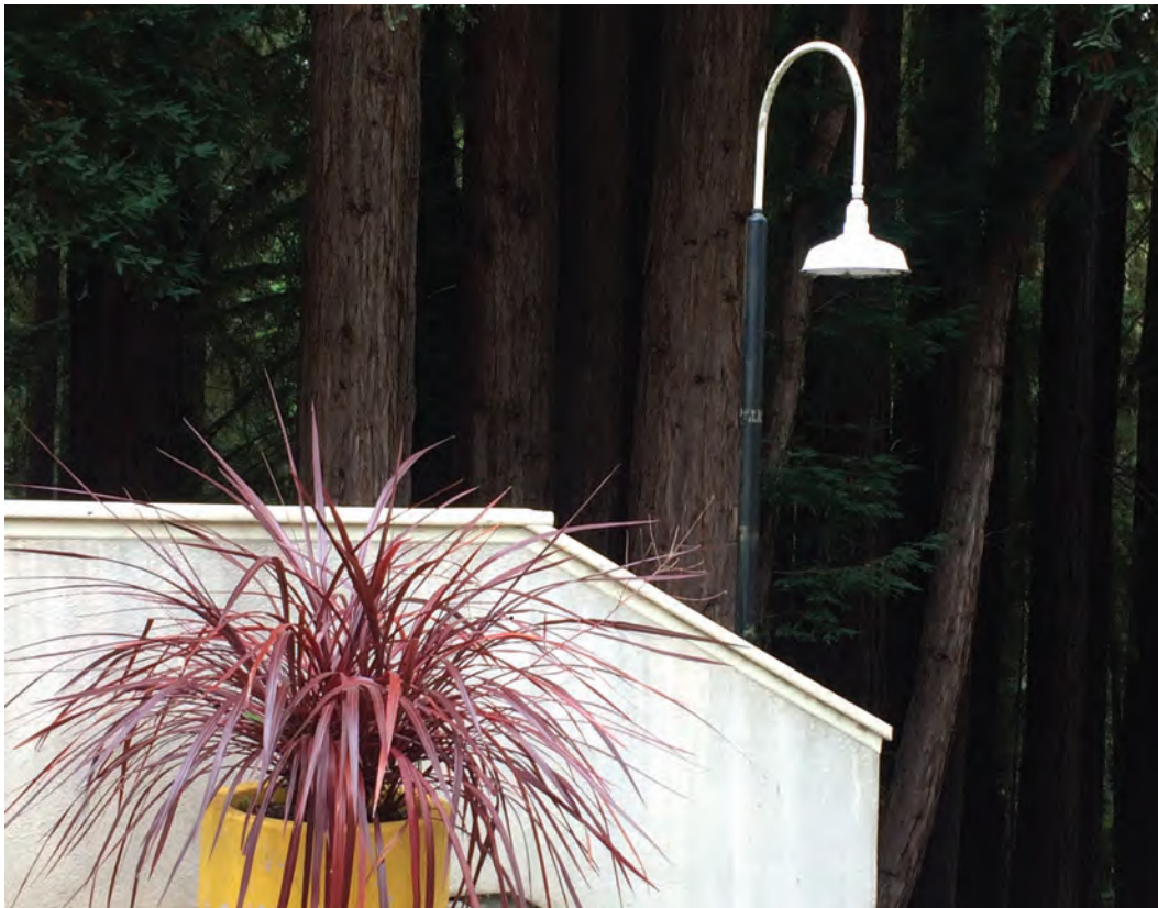
Fig. 3.2.6-10 Existing pole lighting
