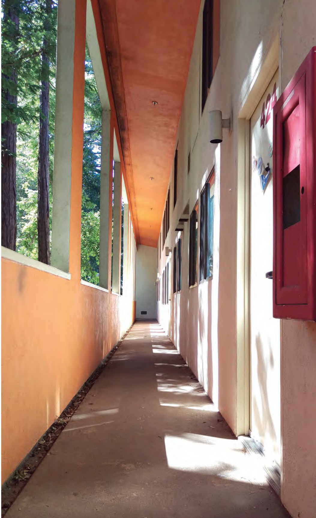
Fig. 3.2.3-3 Second floor entries off cantilevered walkway with Screen Wall with continuous linear trench drain (R4)
