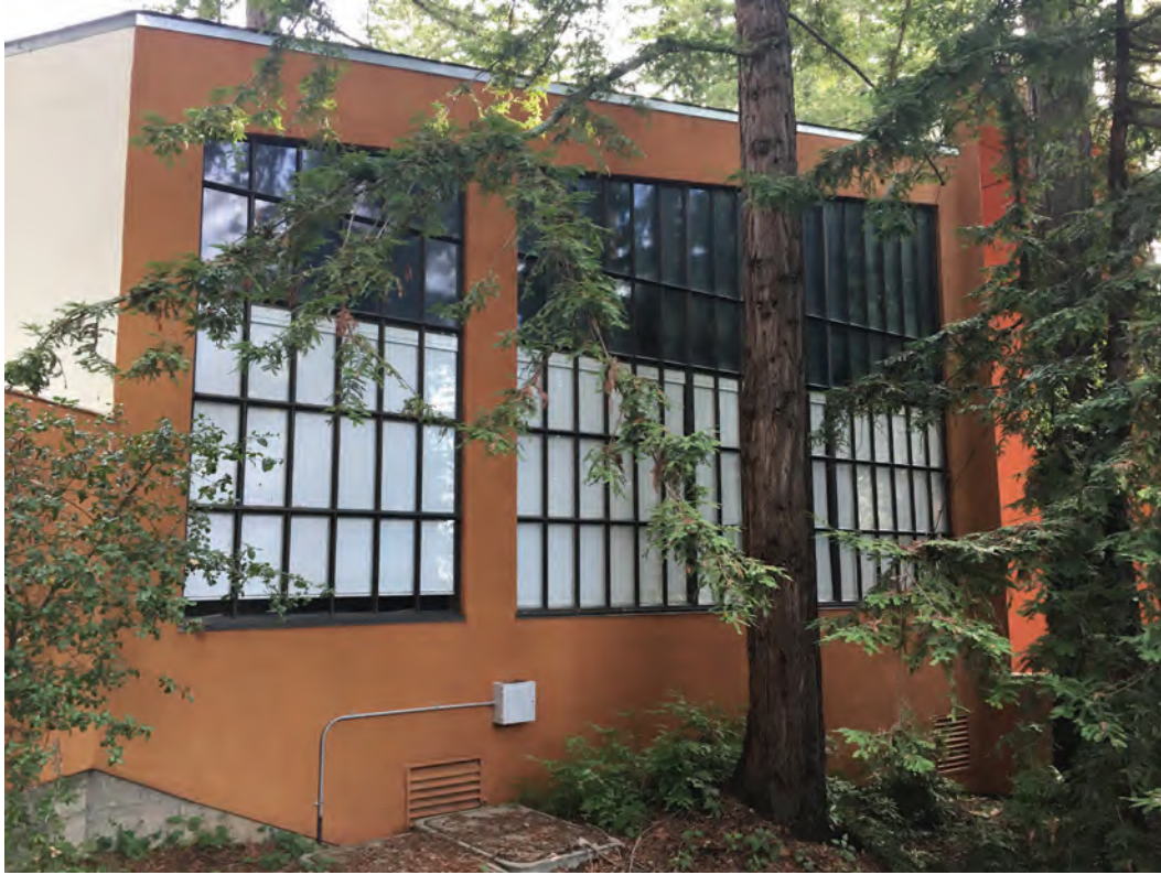
Fig. 2.2-9 Landscape-facing facade with multi-lite windows
