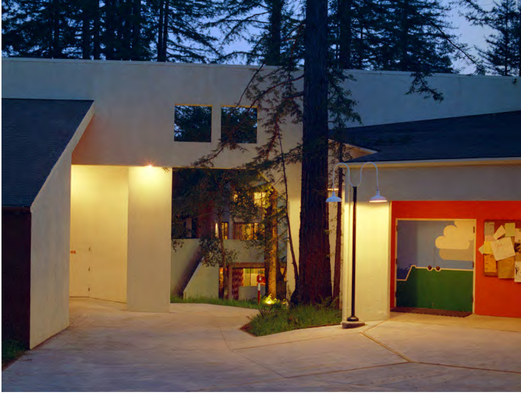
Fig. 4.1.6-1 Wall openings and roofs (Left: G2), doors (Right: A2) (Kresge College, Morely Baer Photographs - UCSC) Archives)
