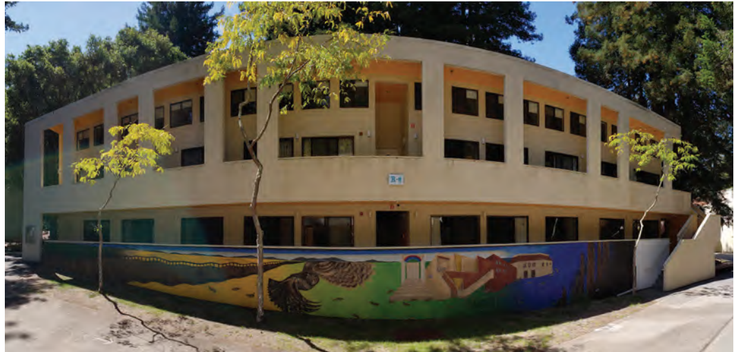
Fig. 3.2.2-5 Existing windows types and alignments (R6)
