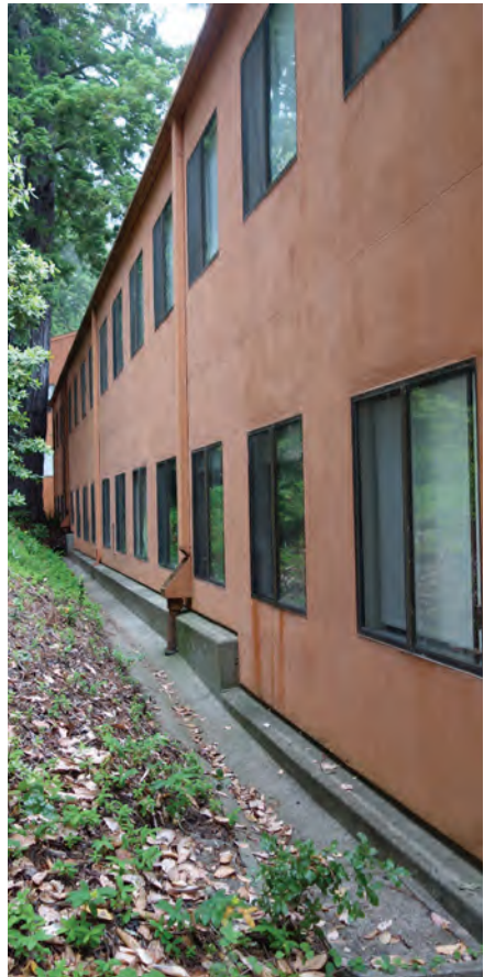
Fig. 3.2.5-2 Existing condition of downspouts and gutters at rear of building (Left & Top: R1, Bottom-Right: R6)
