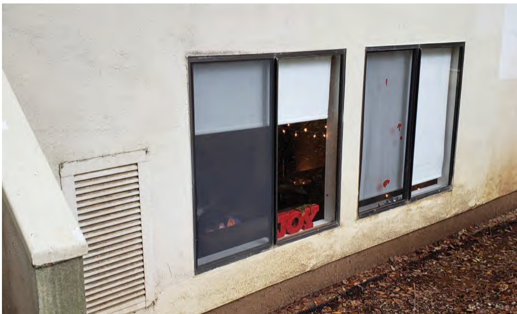
Fig. 3.2.5-5 Existing windows (R4)
