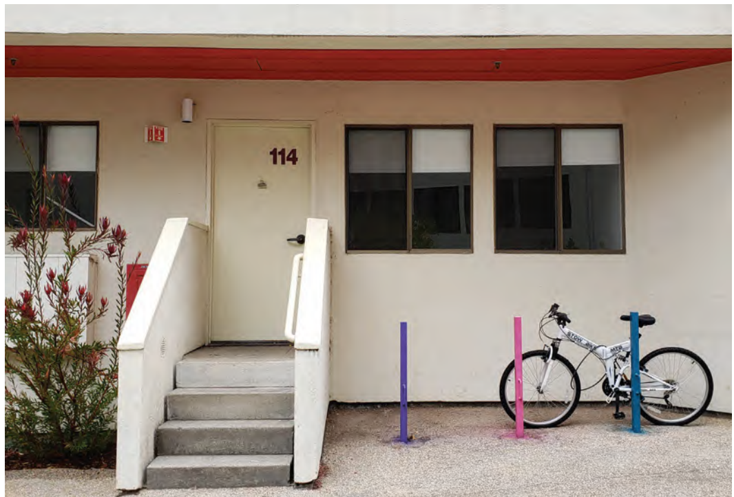
Fig. 3.2.3-2 Existing first floor entry stoop (R1)
