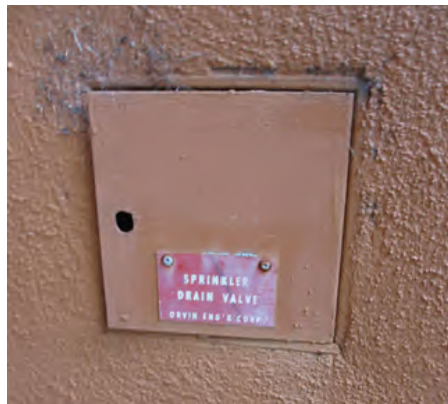
Fig. 3.2.5-8 Existing access panels and vents painted to match the facade color (R2)
