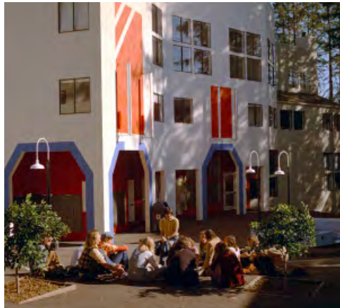
Fig. 4.1.6-1 Wall openings and windows (A1) (Kresge College, Morely Baer Photographs - UCSC) Archives)
