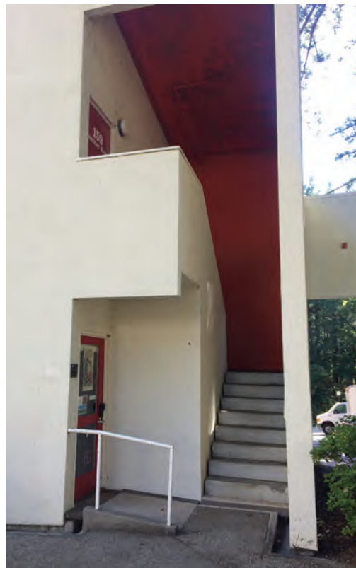
Fig. 2.2-22 Accent colors at upper level covered walkway, north-west stair, and doors
